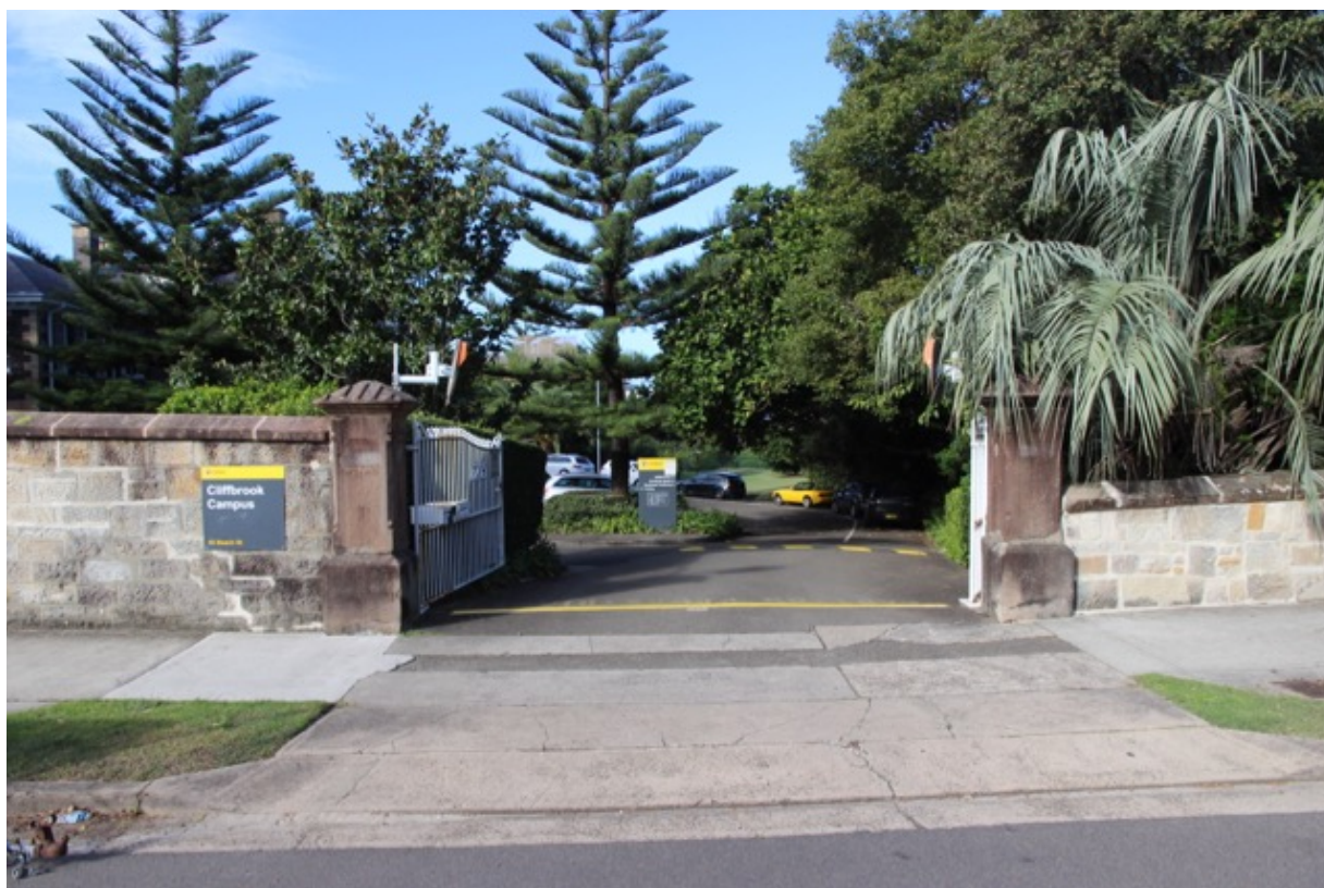
Figure 56: CliffBrook Campus (main entrance & driveway)
