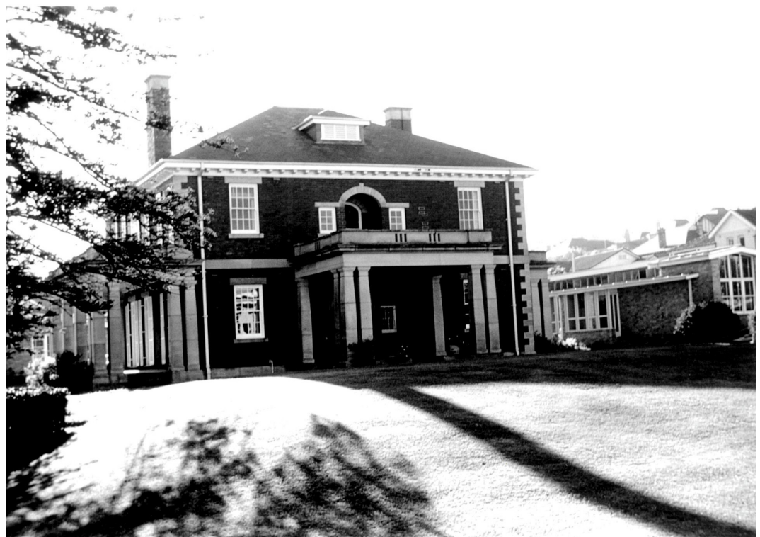
Figure 43: Cliffbrook with CC2 offices building adjacent (Nd)
