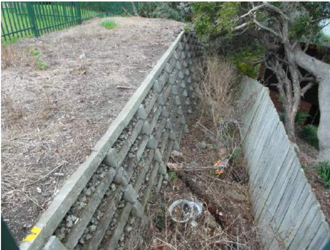
Figure 10. View south-east over built up retaining wall containing piped drainage.
