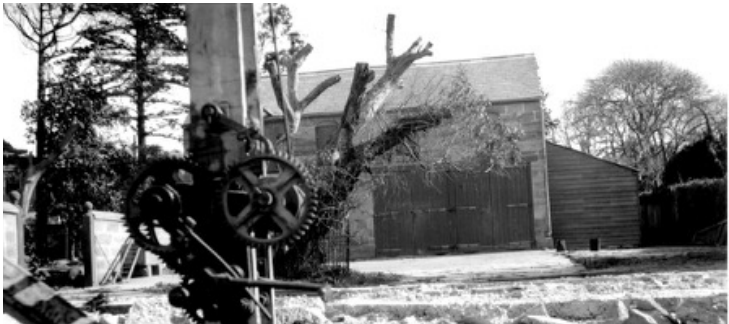
Cliffbrook under Construction - Stable buildings in the northwest corner of the study area (c.1921/22)
