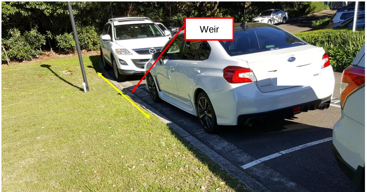
Figure 17 – Overland flow weir downstream of the Site vehicular entrance
