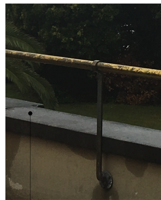
6 DETAIL Photo - Existing Handrail
