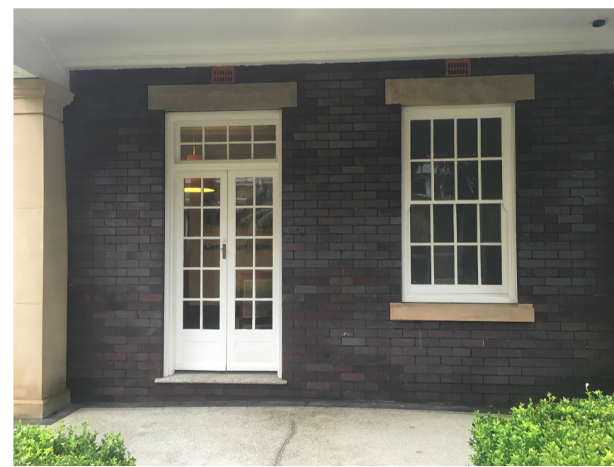
1 DETAIL Photo - Existing Elevation
