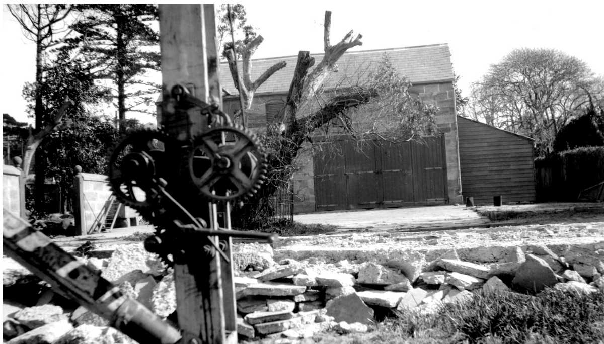
Figure 38: Cliffbrook under Construction - Stables complex buildings in the northwest corner of the study area (c.1921/22)
