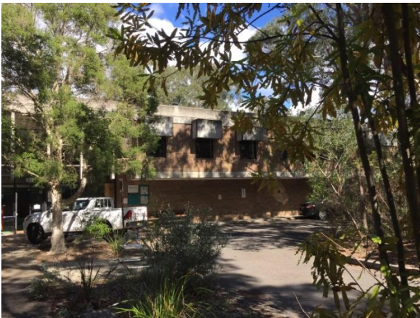
Picture 7 – External view of existing building
