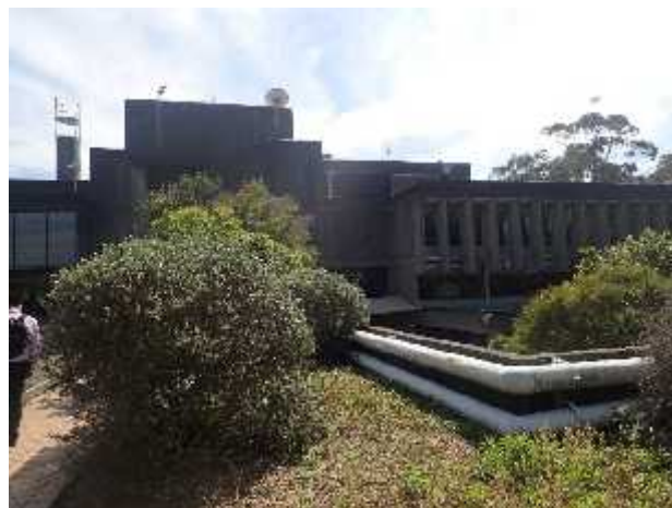
Roof top landscaped planters
