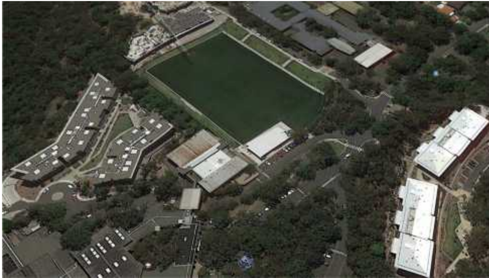
Public open spaces and oval surrounding the existing building
