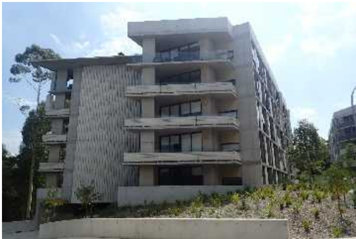
5 storey residential blocks to the West of the former UTS Ku-ring-gai campus
