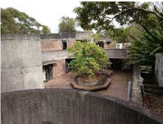
Stepped roof terraces
