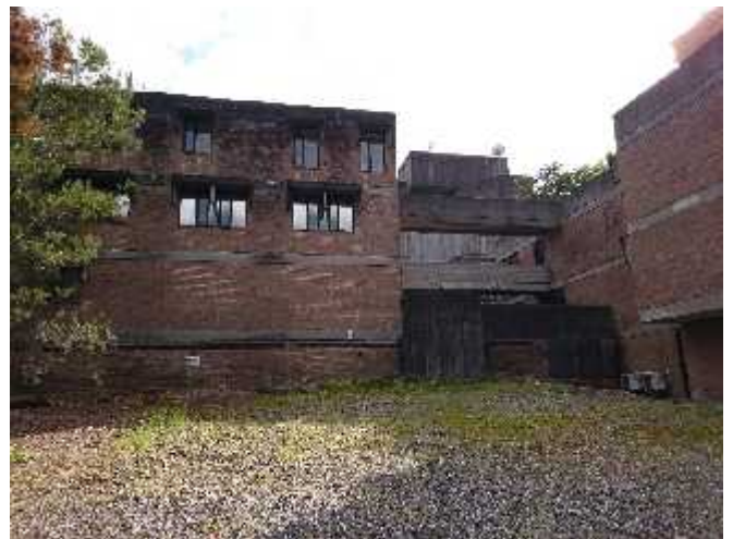
Fenestration 1800mm high with narrow sashes
