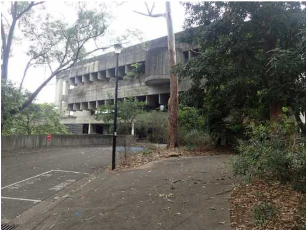
Former UTS Ku-ring-gai Campus view from the East
