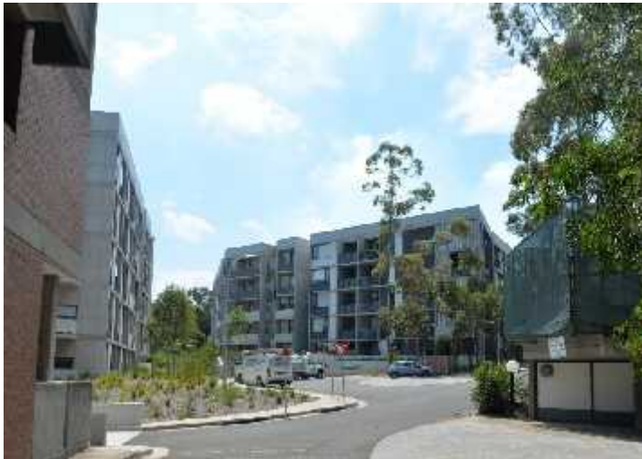
5 storey residential blocks to the West of the former UTS Ku-ring-gai campus
