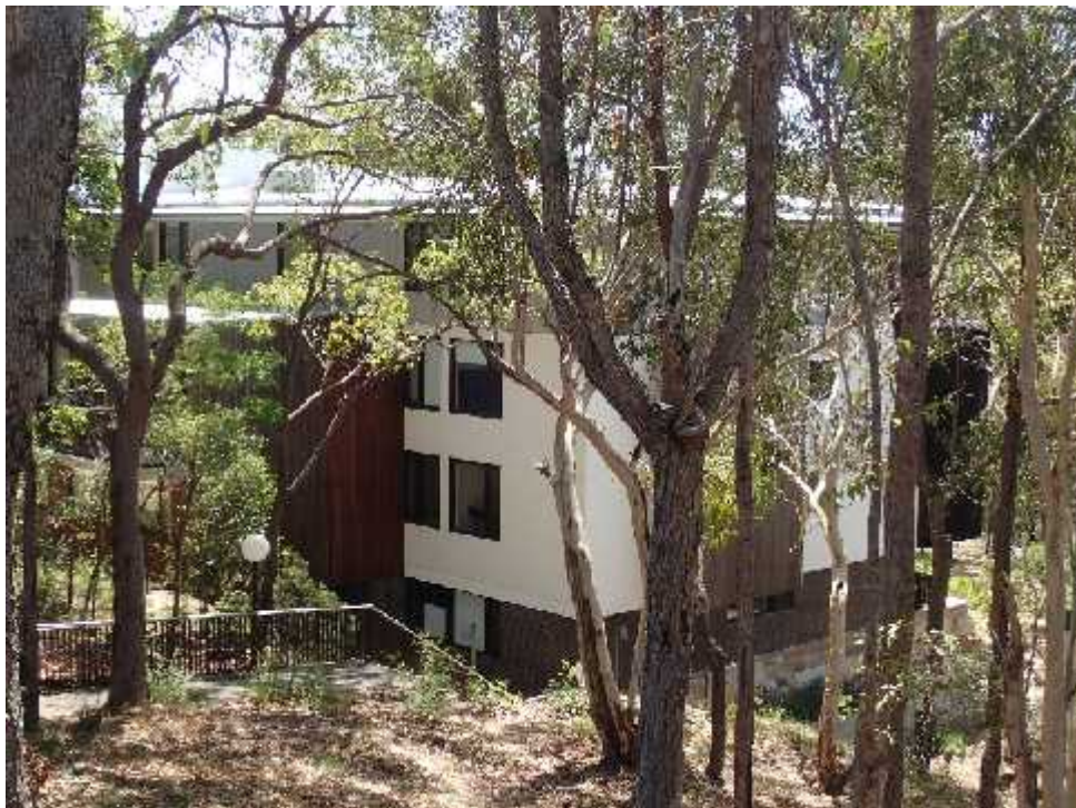
4 storey residential blocks to the North of the former UTS Ku-ring-gai campus
