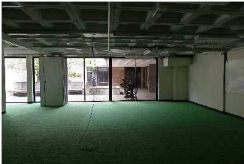
Existing classrooms to be refurbished into General Learning Spaces
