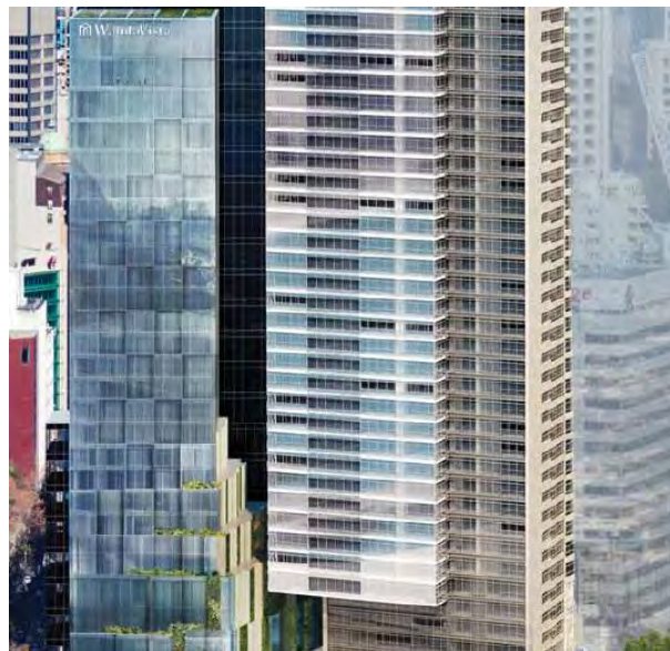
Picture 20 – Wanda Vista Top of Building Signage
