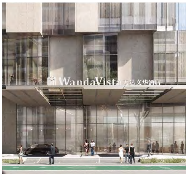
Picture 19 – Wanda Vista Top of Awning Signage
