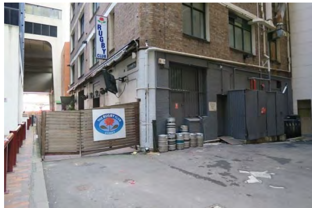
Picture 5 – View of the ground floor of the Rugby Club facing northwest from within Rugby Place
