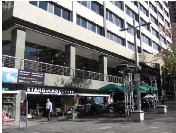
Picture 8 – 1 Alfred Street Forecourt
