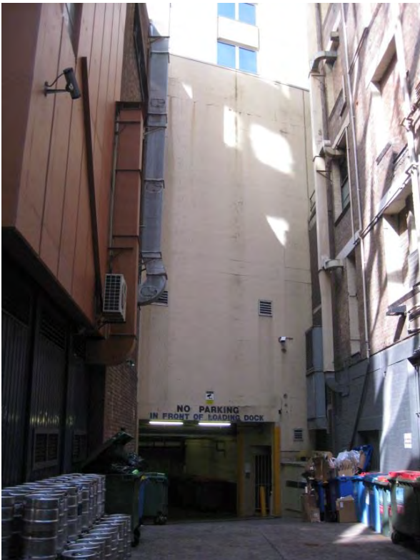
Picture 13 – Rear Access and Loading Bay Dock to the South of 1 Alfred Street
