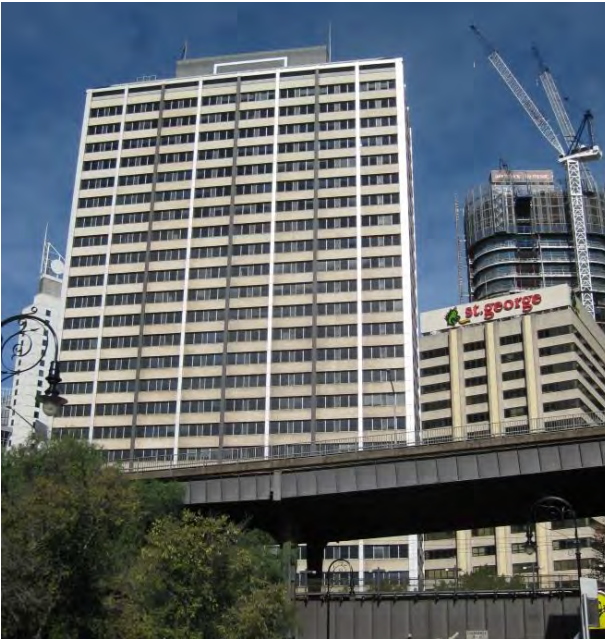
Picture 1 – View From The North
