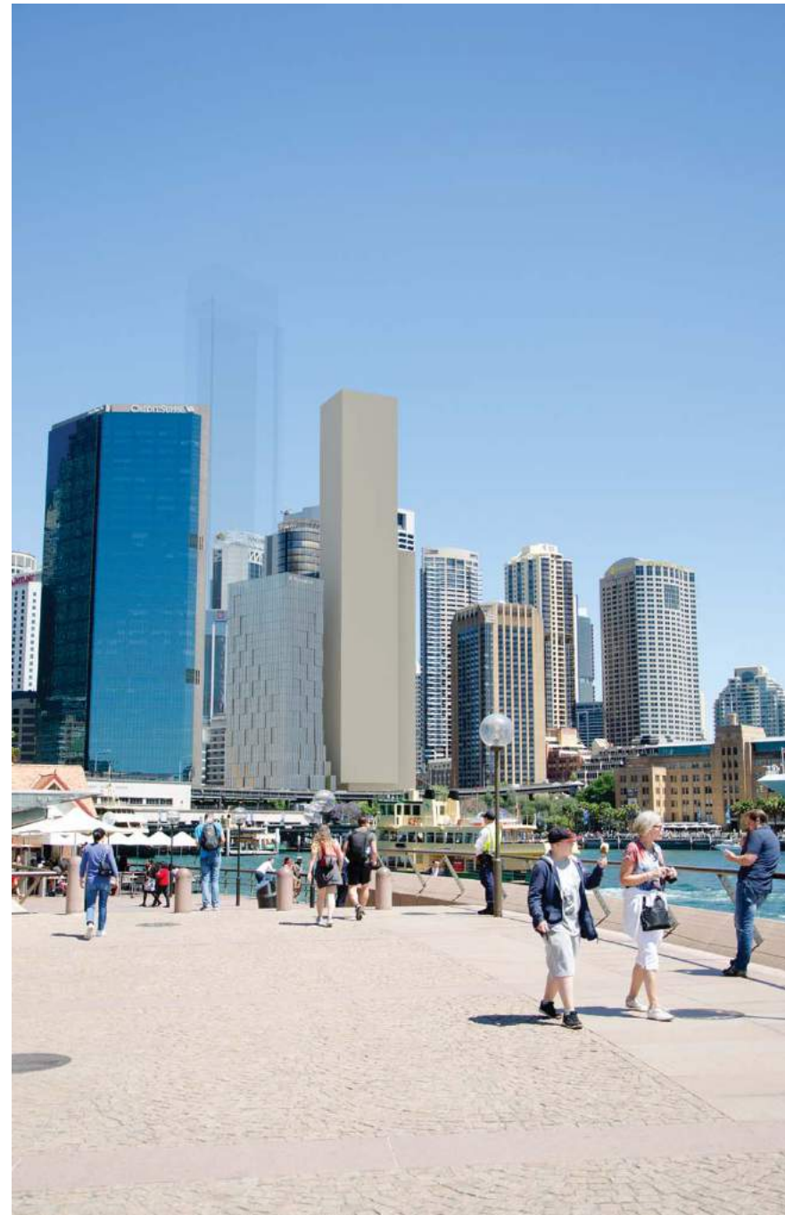
B1: Opera Bar - Looking South
