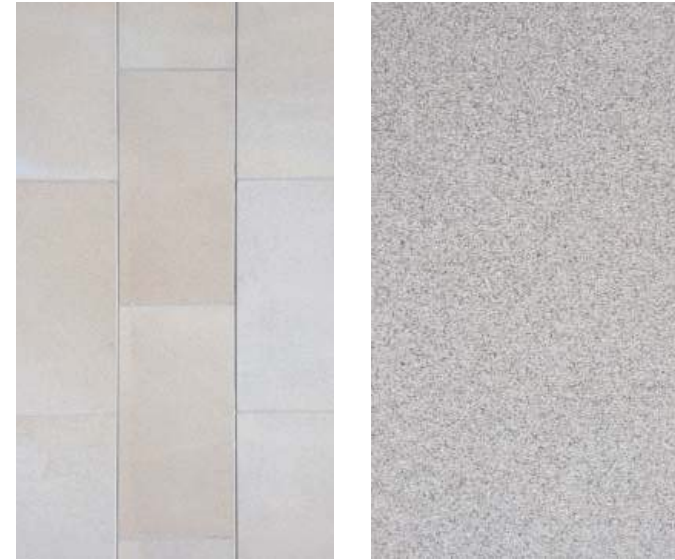
Sandstone | GFRG Relating the building to contemporary and historical buildings. Sandstone to Ground, GFRG above Ground level
