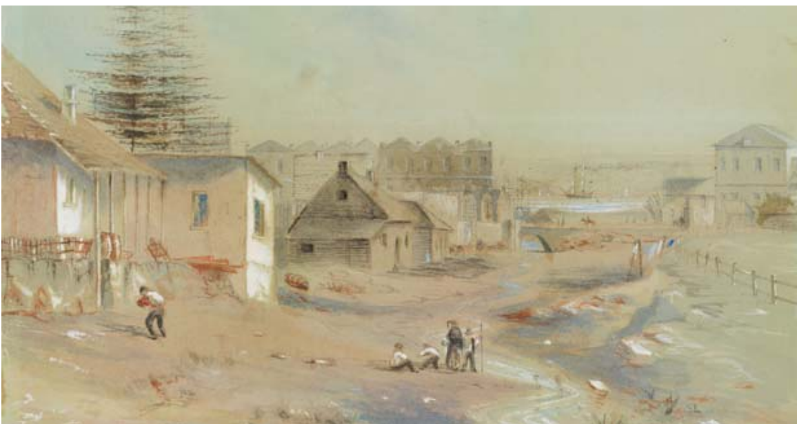
Figure 17 – Frederick Garling's 1842 watercolour shows the Tank Stream, emptying to Sydney Cove
