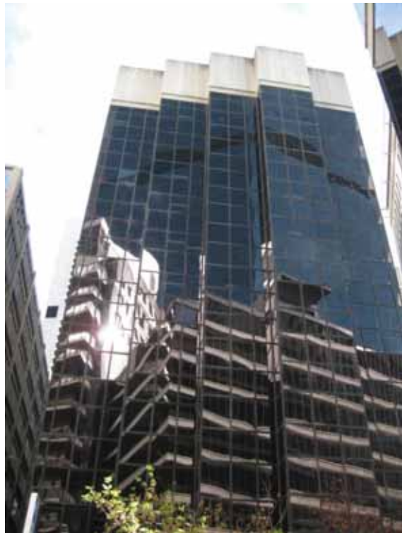
Picture 12 – 33 & 35 Pitt Street
