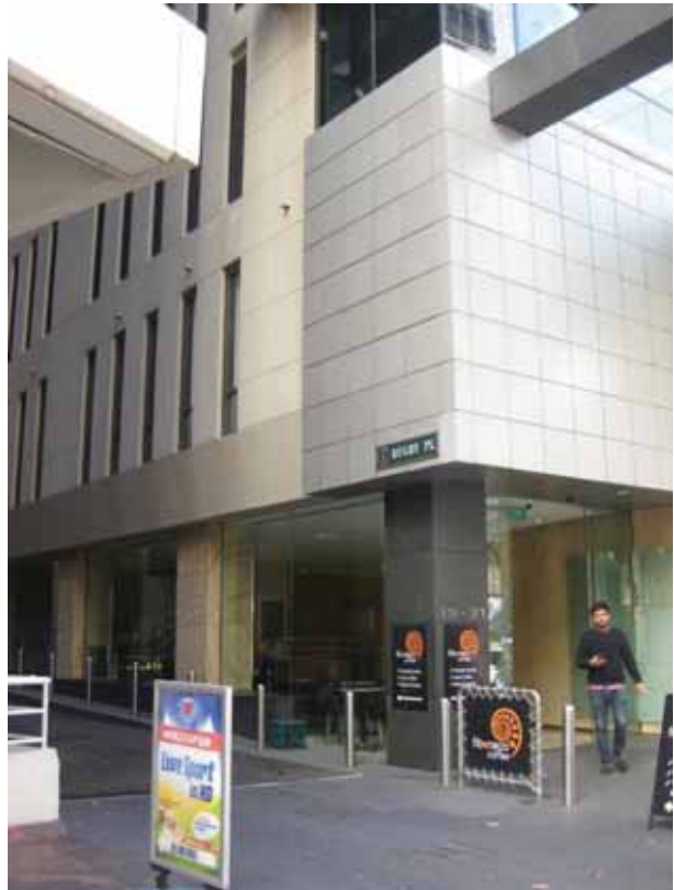
Picture 4 – Pedestrian Access To 19-31 Pitt Street from Rugby Place
