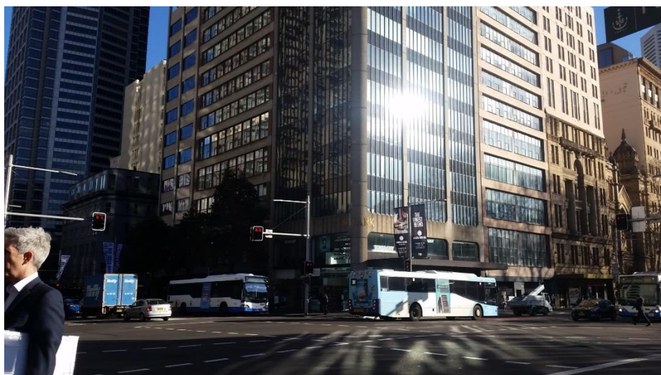
Figure 16 – Surrounding development – Park Street Source: JBA
