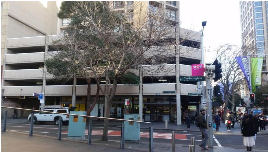
Figure 18 – Surrounding development – Park Street Source: JBA
