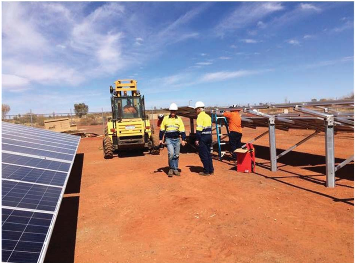
Plate 2: Module Assembly
