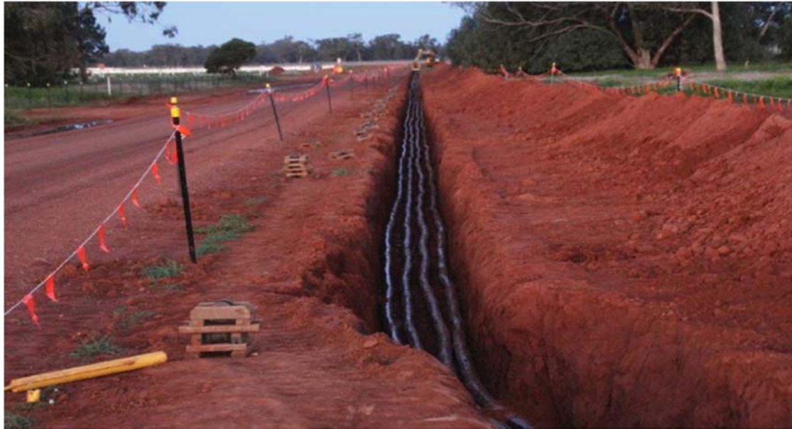
Plate 3: Typical cable trench for MV collection system
