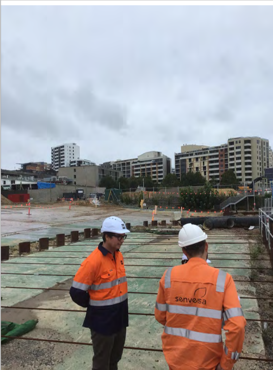
Photo 3: Sheet pile wall and anchors
