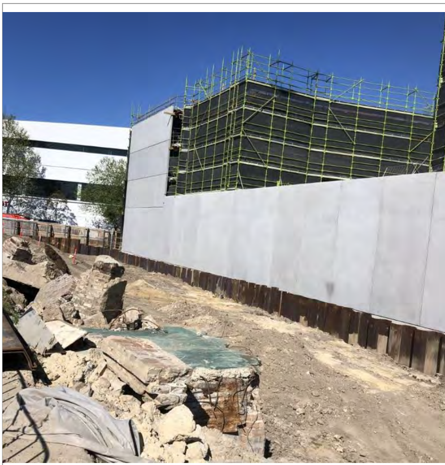
Photo 9: Looking south-east from southern portion of Stage 2. Sheet pile walling has been installed along southern boundary of Stage 2 to prevent off-site migration. Groundwater extraction is also occurring along this boundary.
