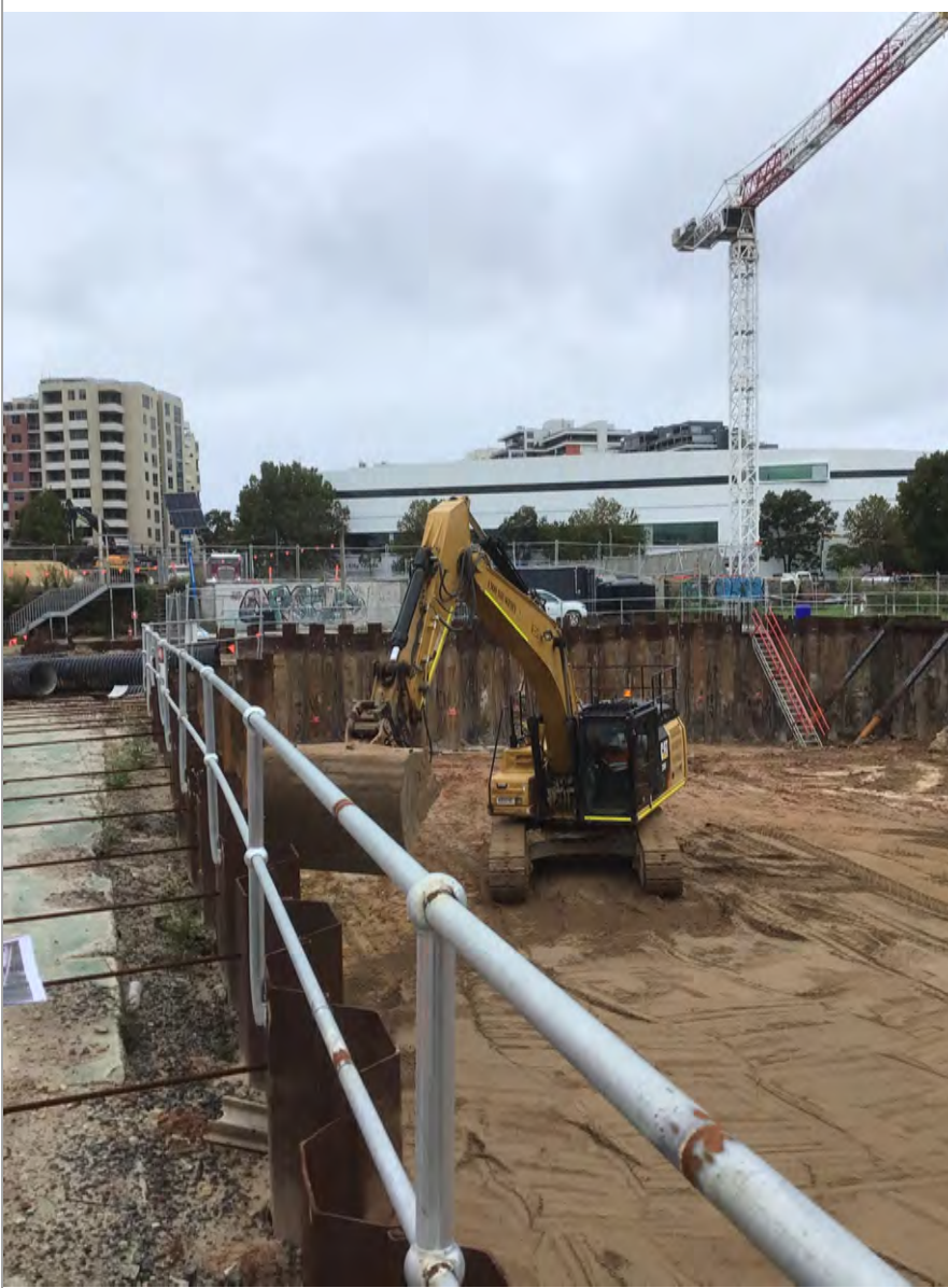
Photo 1: RA2 – placement and compaction of remediated Botany Sands
