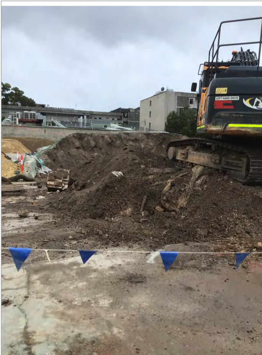
Photo 6: Stockpiled material in stage 1 contains bonded asbestos. Being taken off-site to landfill as GSW special waste.
