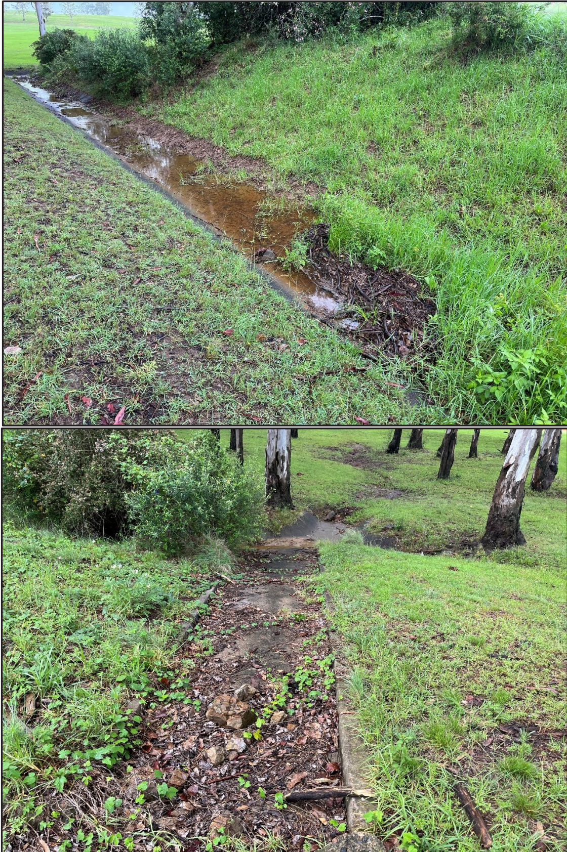
Figure 8 MZ3 Current Condition
