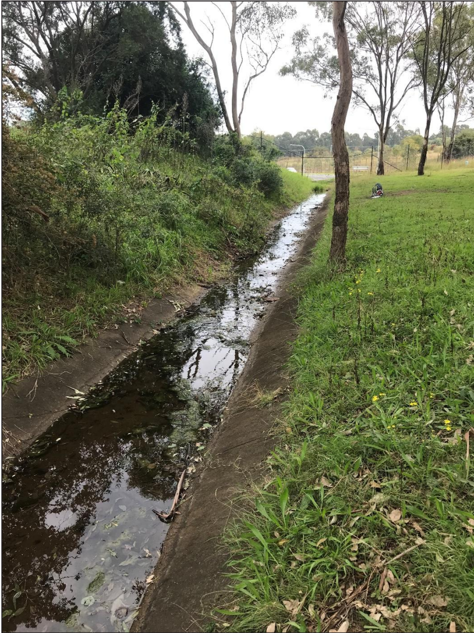
Figure 14: Concrete drain mapped as 1 st order stream within the development footprint
