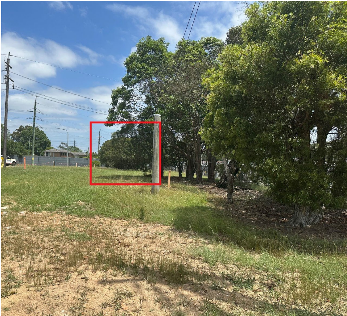
Photo 2-5: Looking west onto Old Windsor Road showing noise wall with vegetation identified for removal and nearest sensitive receiver.
