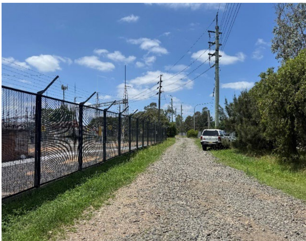
Photo 2-1: Looking southeast onto driveway within site
