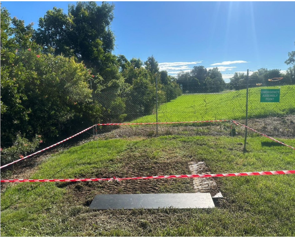
Photograph 19: 2026 View of pipeline corridor looking east from TP07.
