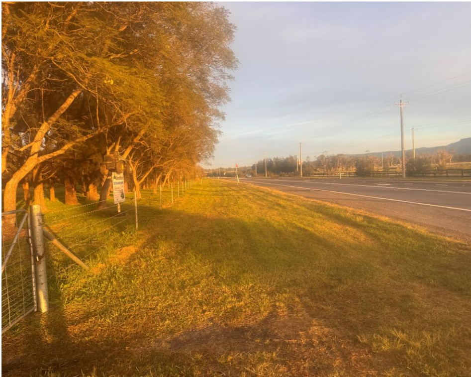
Photograph 1: View of Bolong Road and proposed location of underbore. Borehole BH01 on northern side of road
