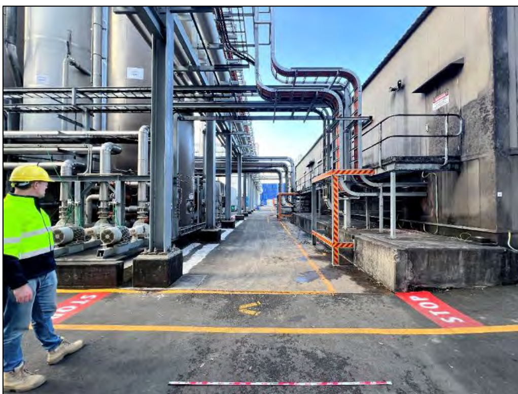
Plate 9: Looking east through existing Manildra infrastructure and proposed pipeline route.
