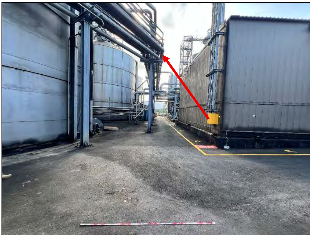
Plate 8: Start location of pipeline route within existing Manildra facility (pipeline will connect to existing raised infrastructure).
