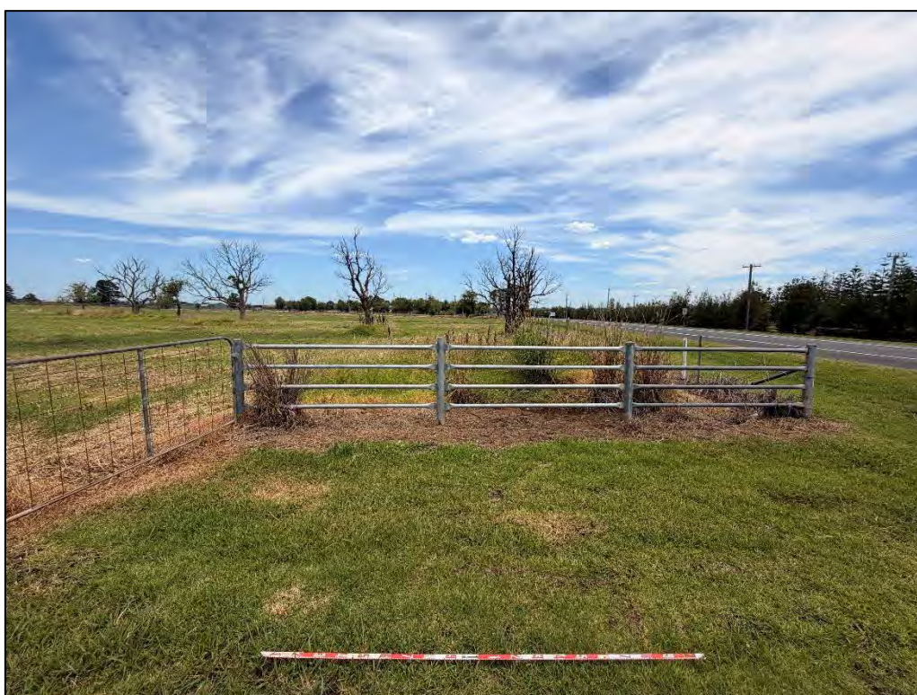
Plate 5: Looking west along proposed pipeline route adjacent Bolong Road.
