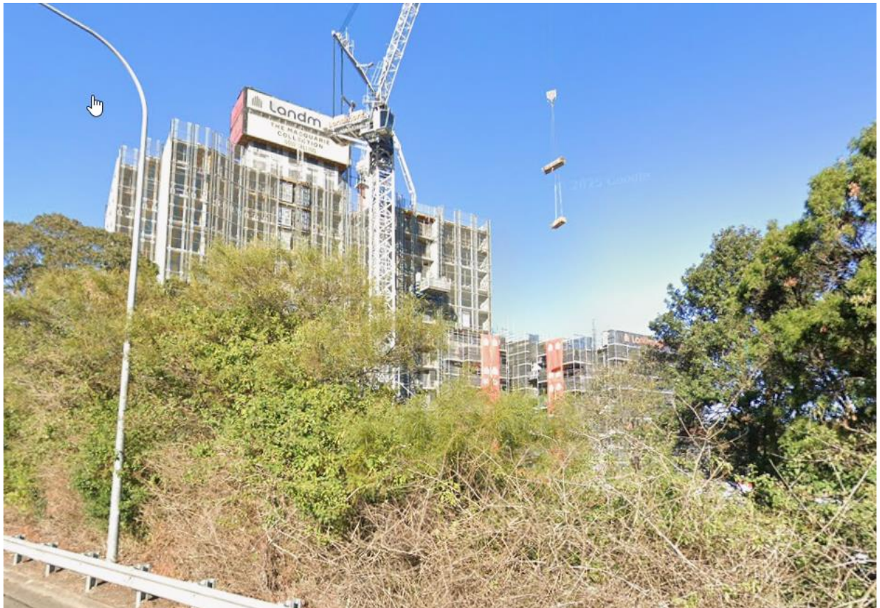
Figure 2: No. 5 Halifax Street, south of the subject site (source: Google Maps view from M2 Motorway - July 2025)
