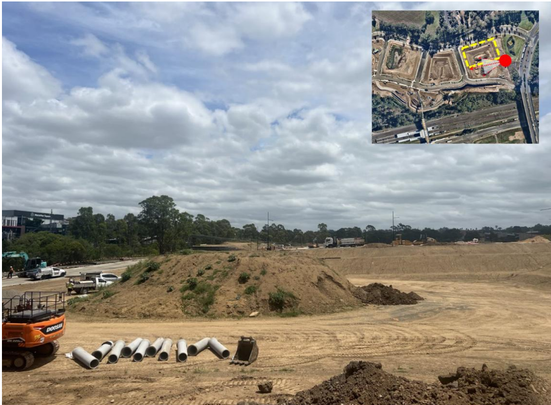
Figure 3: View from east of site looking west (Source: Keylan)
