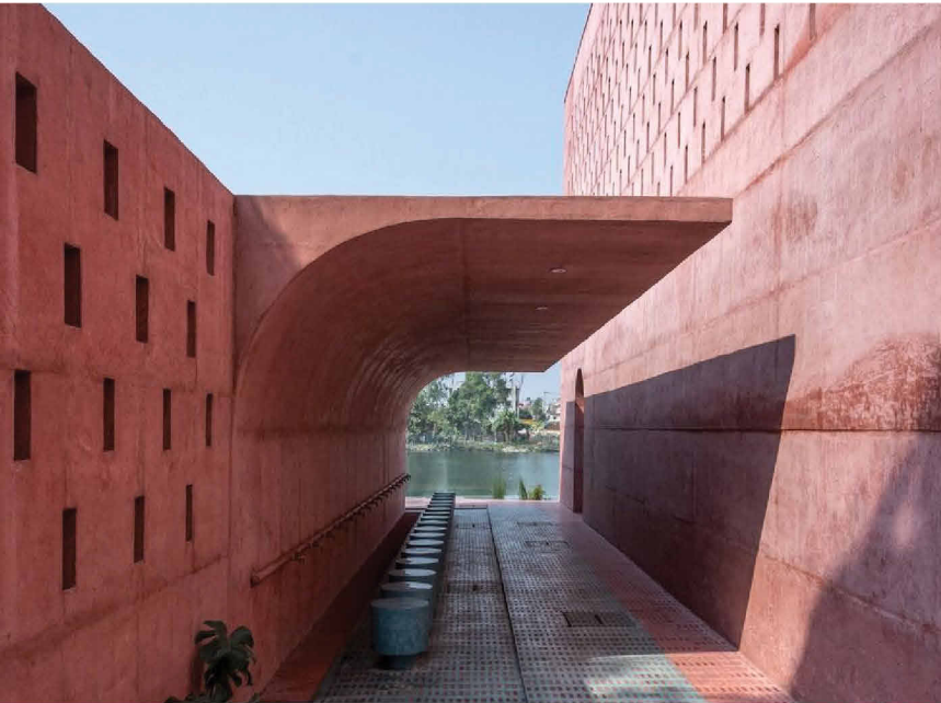
W1 CONCRETE RETAINING WALL
