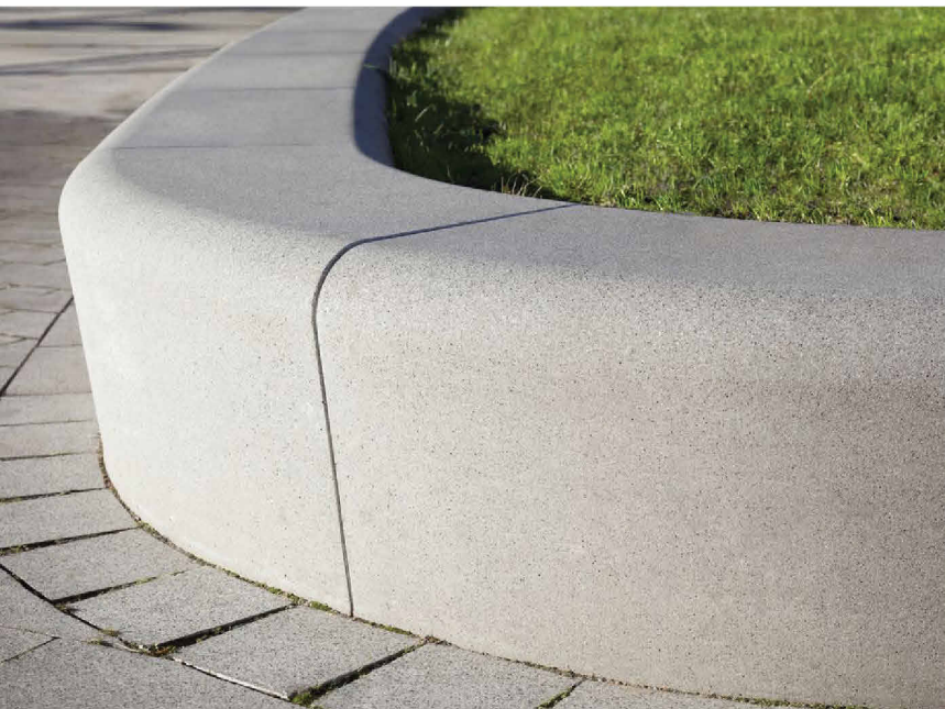
W2 CONCRETE RETAINING WALL
