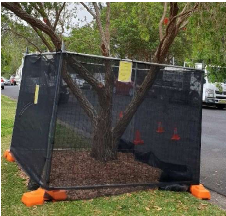
Figure 19 Example photos showing tree protection zone fencing with pad footings and bolt cleated panels, and TPZ signage. The TPZ fence locations are on the Arborist Impact Plan Arb_602.
