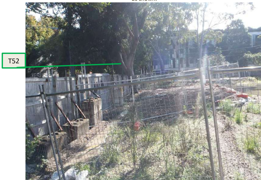
Figure 32. Trees T52 and T51 (Tuckeroo) All have been fenced off with mulch as shown. Note: there appears to be footing/concrete slab remaining within the TPZ of this zone (as described in Chapter 6 c and Figure 5).
