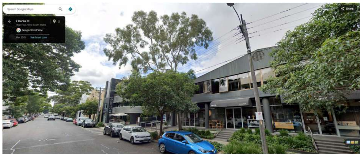
Figure 12. Views looking towards T37. This photo is March 2021 and shows the buildings erect. This photo is useful in showing a fuller canopy condition and density and to show the garden bed within which it was growing in comparison to current photos below in figures 14-16.
