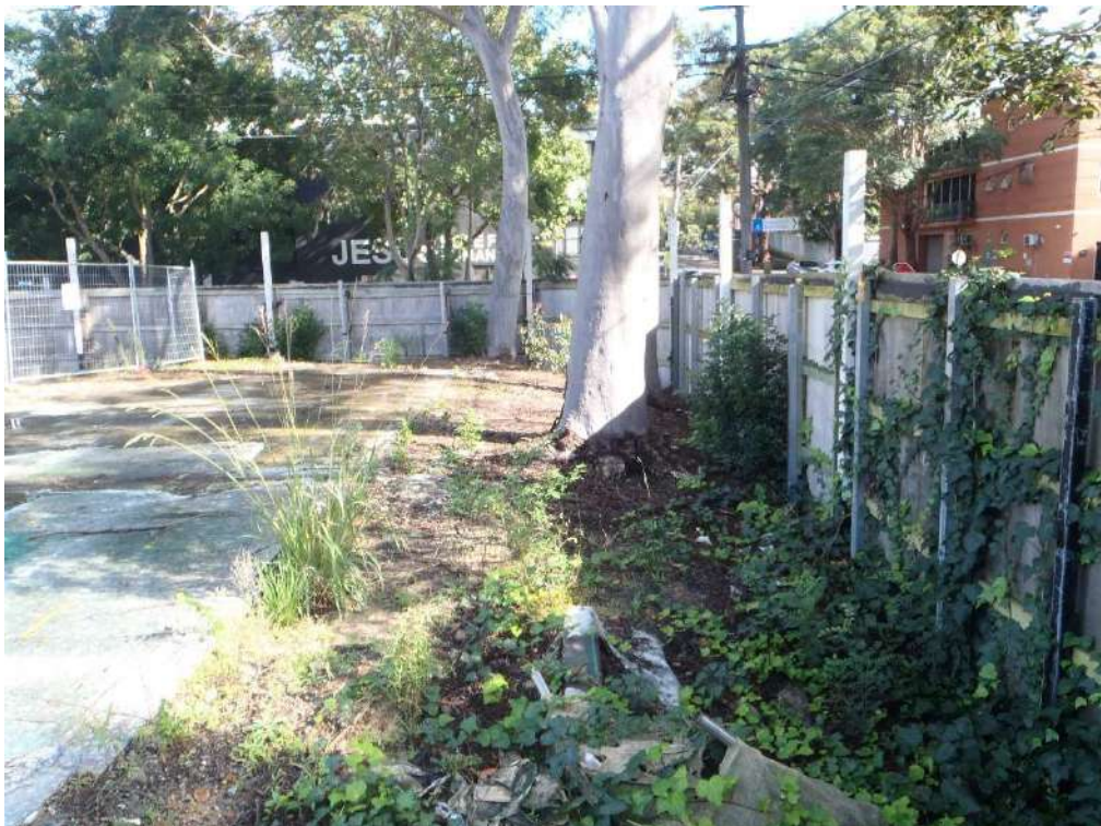
Figure 39. Close up views (both photos) of the trunk and ground condition of T41 (foreground) and T44 (background). Note: T42 and T43 are obscured by the trunk of T41. Photo looking west. Note retained slab (semi-circle) and understood to have the underground arrangement described in Figure 5. Retain TPZ fencing in place for the Main Works DA and for tree stability (utilising the slabs for stability)
