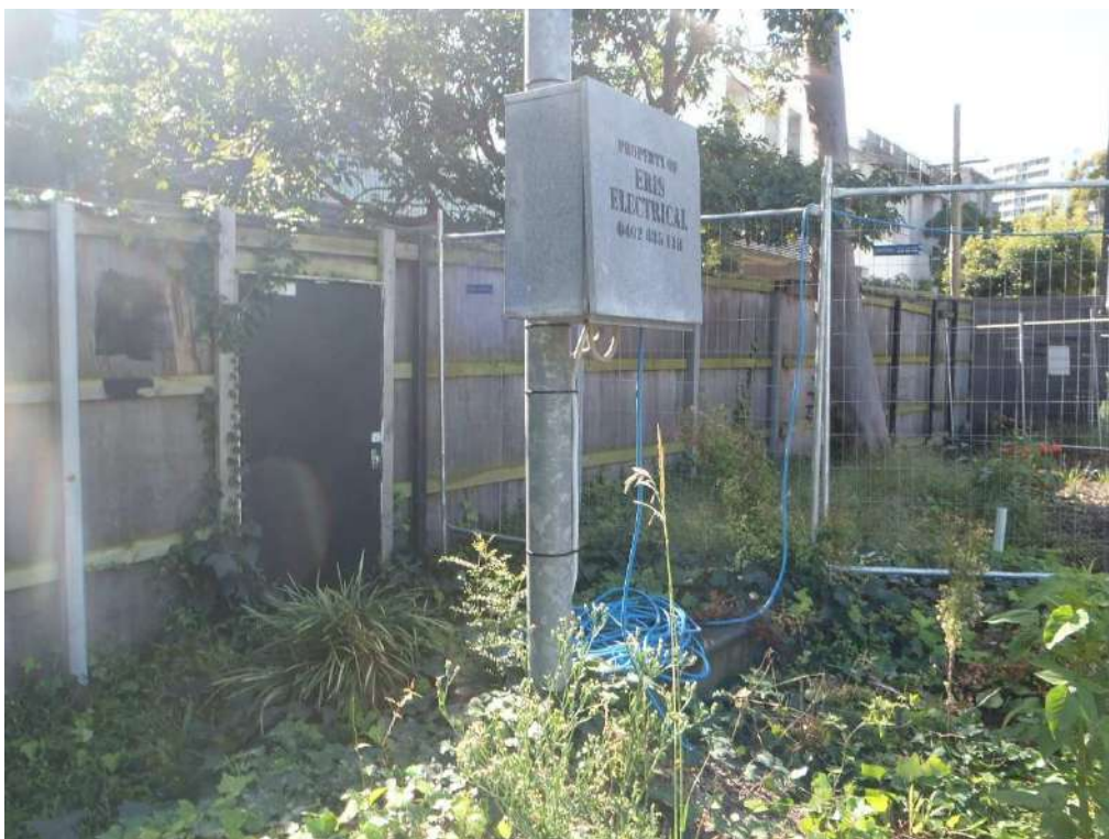
Figure 37. Close up views (both photos) of the trunk of T37. Note the slight lean to the north (towards Danks St). Note also the electrical services box and entry door at hoarding.
