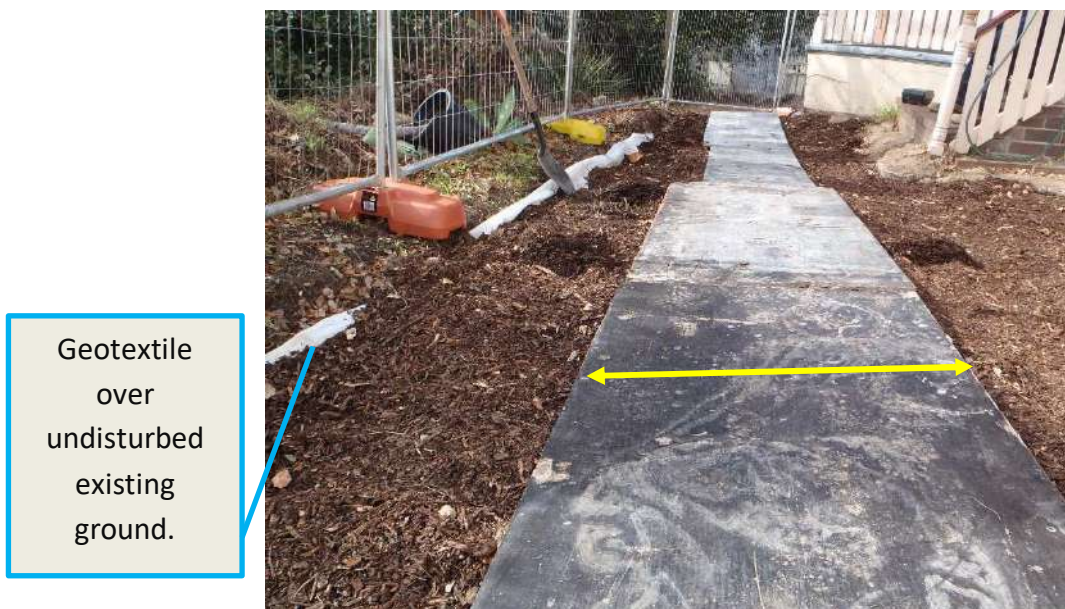
Figure 18 Example photo showing ground protection boards over mulch and over geotextile. Note: mats/boards must meet (no gaps), be fixed together and fill the whole width of the ground protection zone + to the edge of the fencing as depicted on the Arborist Plans.
