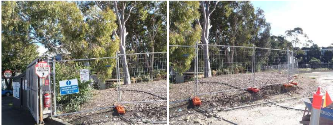
Figure 24. View looking west with Gate 2 Entry on the far left (off Young St). Trees are T66 and T65 (Lemon Scented Gums with white trunks) with trees T65a, T63, T62 and T61 towards the right of the photo and all fenced off. Note: The tree protection zone fencing and the mulch zone is slightly larger than is proposed for the Main Works DA where the proposed fencing is set at the TPZ extent. Refer to the Arborist plan.
