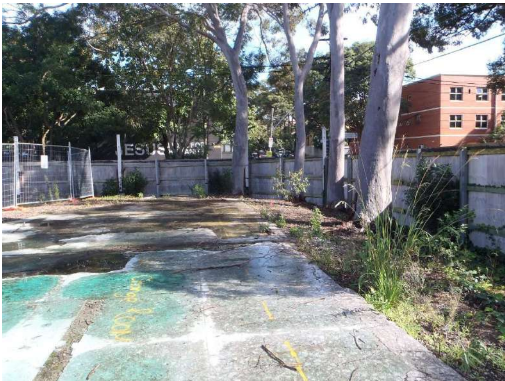
Figure 40. Close up views (both photos) of the trunk and ground condition of T41 (foreground) with T42, T43 and then T44 (in background). Photo looking west (Danks St on right and Young Street straight ahead). Note retained slab (semi-circle) and understood to have the underground arrangement described in Figure 5 (Chapter 6). Retain TPZ fencing in place for the Main Works DA / construction phase and for tree stability (utilising the slabs for stability)
