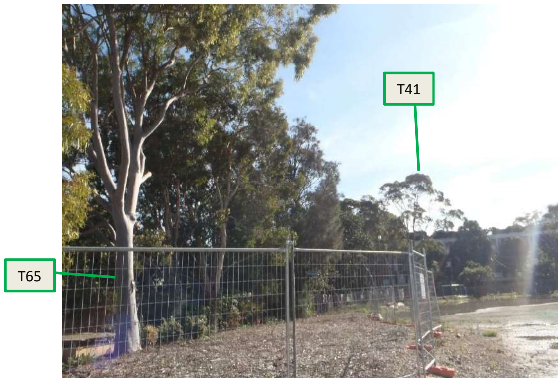
Figure 25. View looking north-west with tree T65 (Lemon Scented Gum with white trunk) with trees T65a, T63, T62 and T61 beyond and towards the centre of the photo and all fenced off. Note: The tree protection zone fencing and the mulch zone is slightly larger than is proposed for the Main Works DA where the proposed fencing is set at the TPZ extent. Refer to the Arborist plan.
