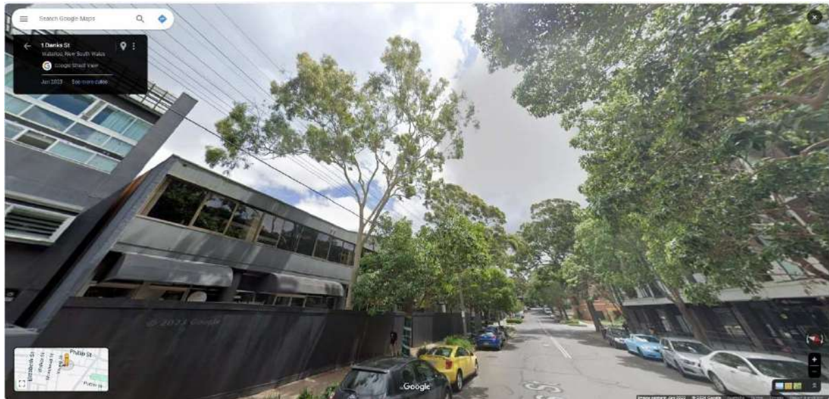
Figure 13. Views looking west along Danks Street with T37 on the left side. This photo is January 2023 and shows the buildings erect and hoarding erected. This photo is useful in showing the canopy condition and density.
