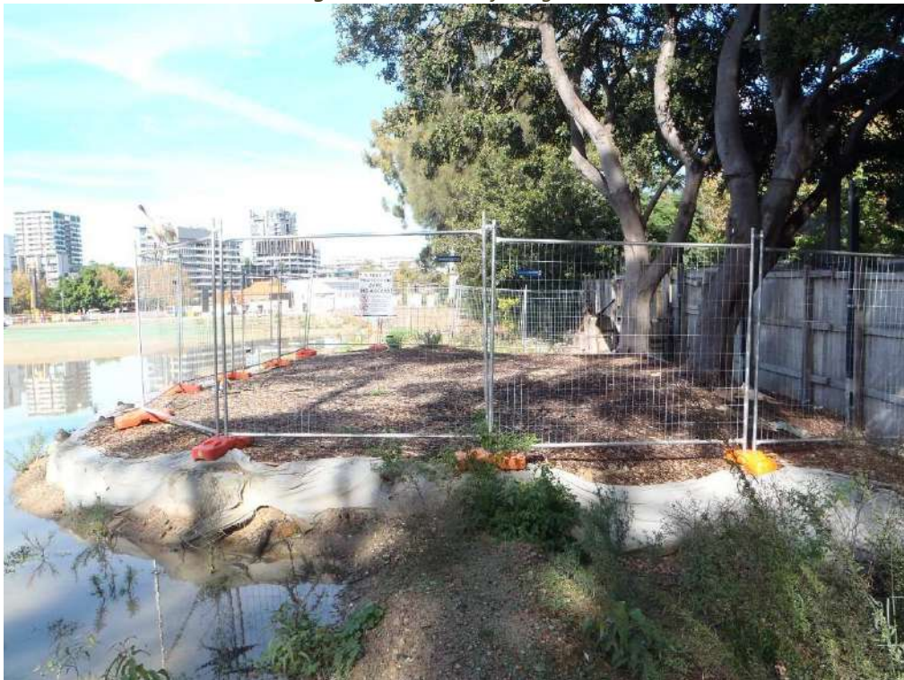
Figure 43. Photo is looking south with T51 and T52 fenced off (Young St to the right). Note there are indications of concrete column footings near the root crown base of these trees and possible slab and understood underground in the arrangement described in Figure 5 (Chapter 6). Retain TPZ fencing in place for the Main Works DA / construction phase and for tree stability (trees utilising the slabs and footings for stability)
