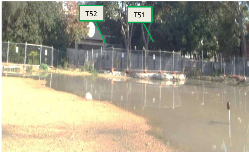
Figure 35. Both photos above are taken from the site looking north-west towards trees to be retained. The recommendation is to retain the already installed TPZ fencing around T37 and T4-T44 and T51 and T52 for the Main Works DA and construction phase. Additional requirements will be needed for future proposals such as for building works and associated landscape design proposals. Trees T37, T41 – 44 and T51 and T52 are all fenced off with mulch and there appears to be footings/concrete slabs remaining within the TPZ of these zones (as described in Chapter 6 and Figure 5), however the extent of concrete for T37 and T51 and T52 is not entirely apparent as mulch is over the top.
