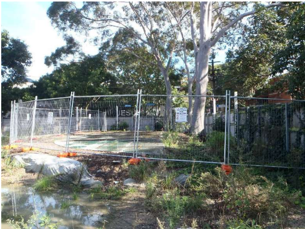
Figure 38. Close up views (both photos) of the trunk of T41. Photo looking west. Note retained slab (semi-circle) and understood to have the underground arrangement described in Figure 5. Retain TPZ fencing in place for the Main Works DA and for tree stability (utilising the slabs for stability).
