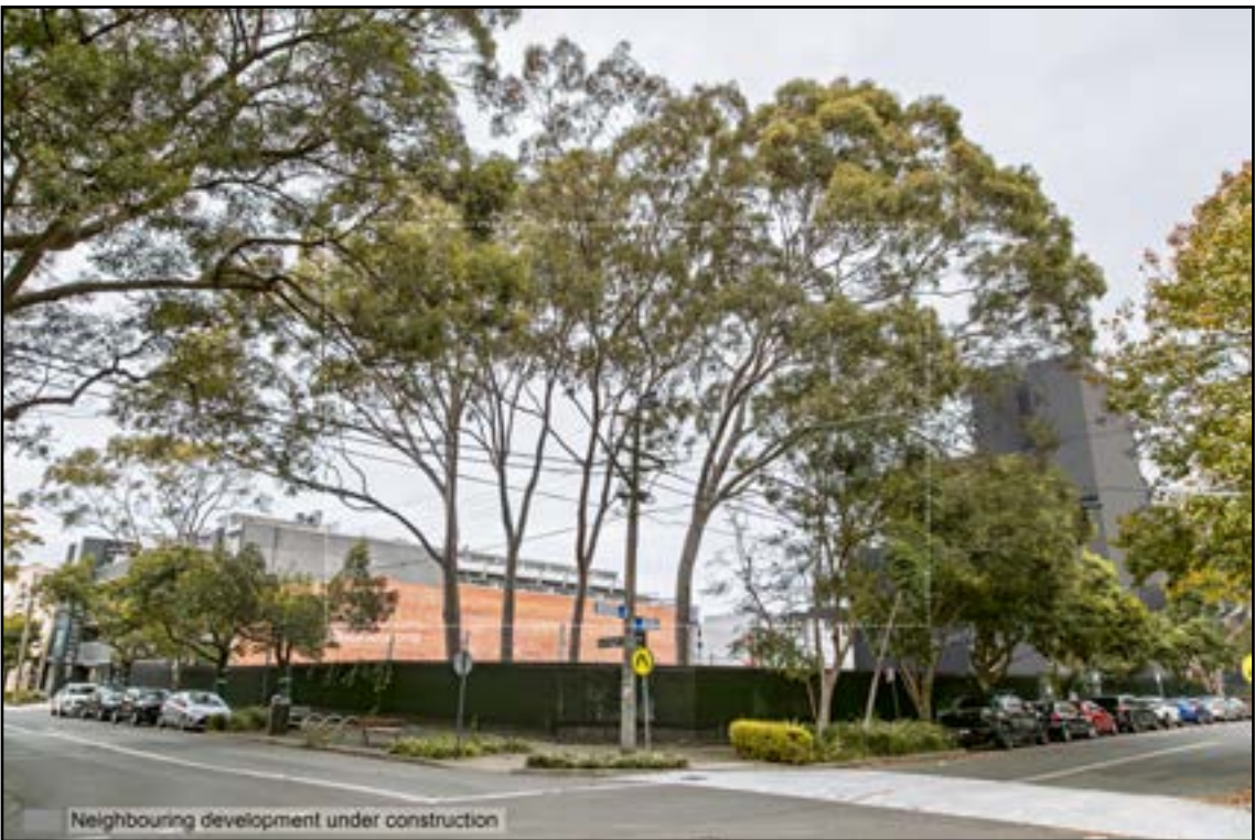
NEIGHBOURING DEVELOPMENT UNDER CONSTRUCTION
