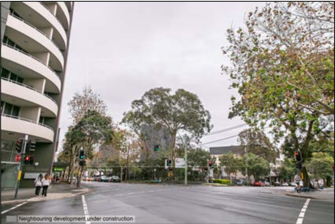
NEIGHBOURING DEVELOPMENT UNDER CONSTRUCTION
