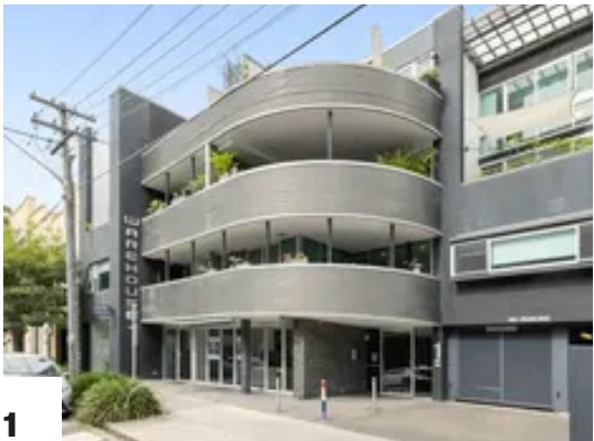
1 Warehouse 1 Danks Street
