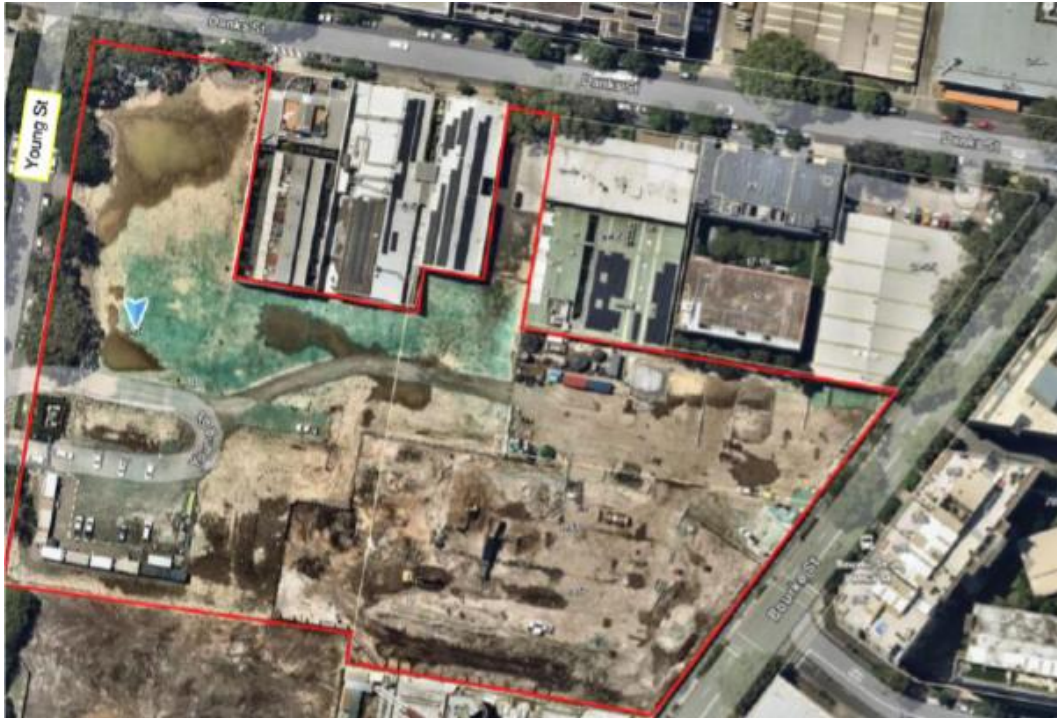
Figure 4.15: Current aerial of the study area showing complete demolition. Source: image supplied by the proponent
