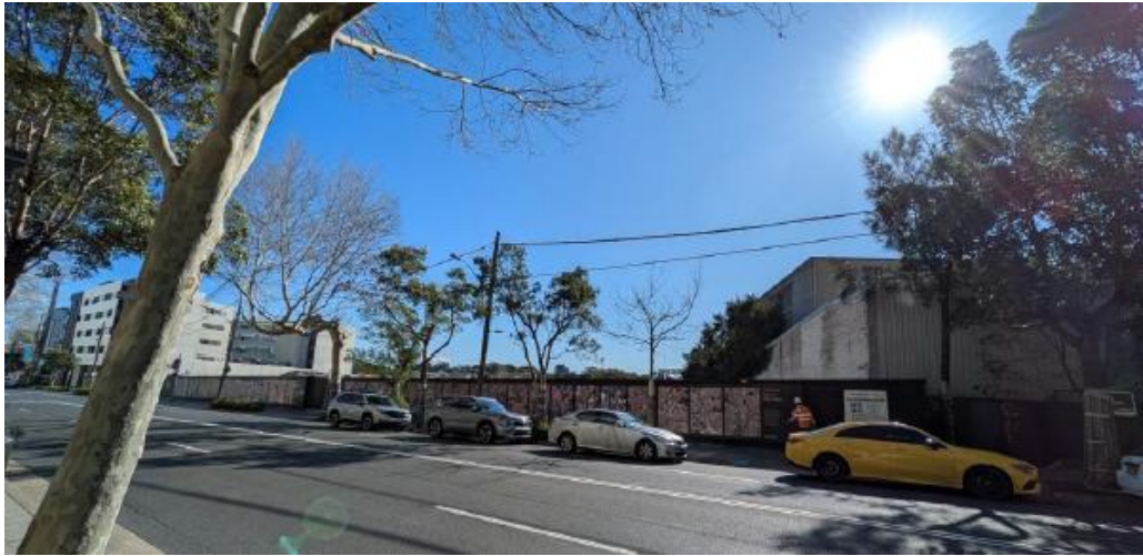
Figure 4.17: View looking towards the study area, from the eastern side of Bourke Street. Source: Curio 2025
