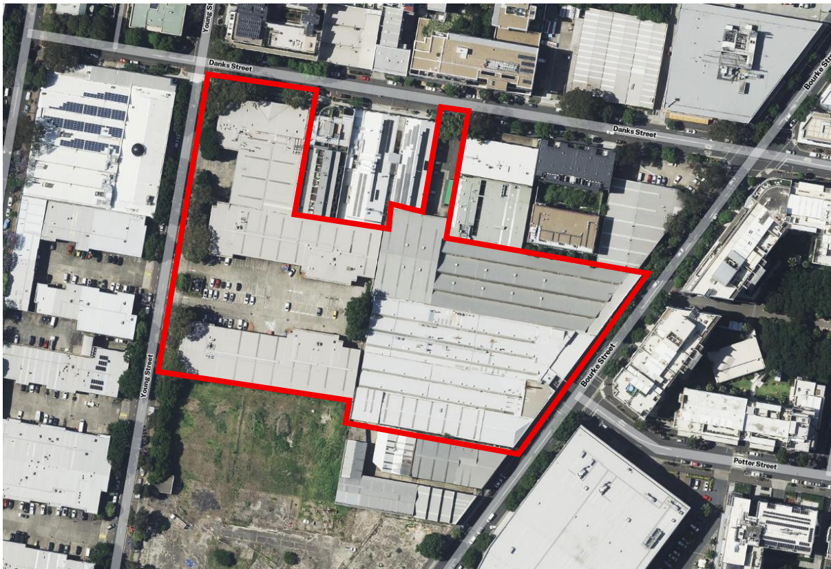
Figure 1.2: Ariel view of study area prior to demolition. Source: Six Maps
