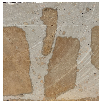
02 Pre-Cast Concrete Panels with Exposed Aggregate
