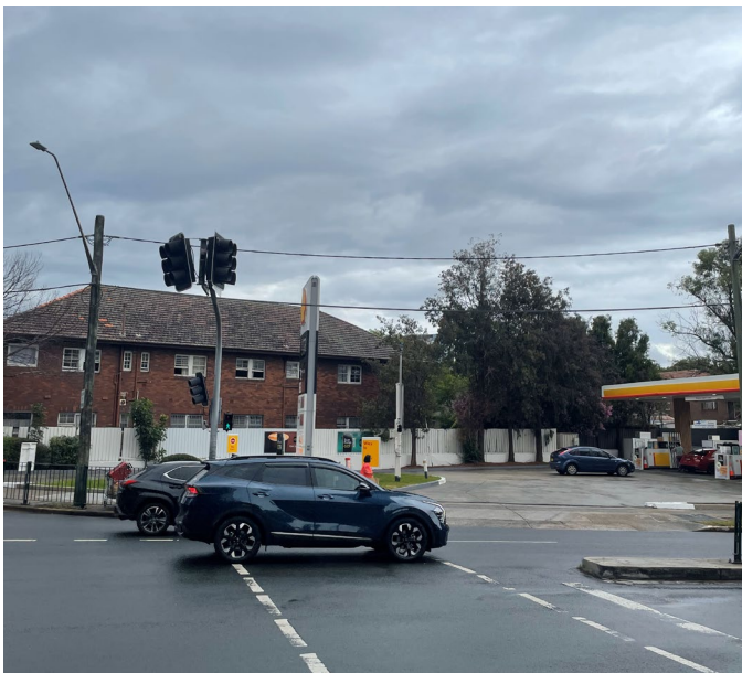
View of 11 Albert Road from Raw Square looking west
