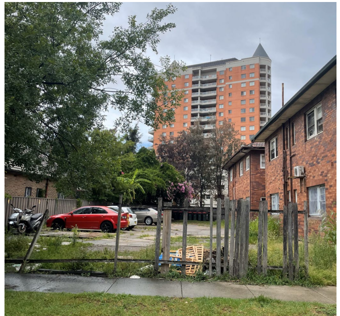
View of the rear of 13 Albert Road looking east
