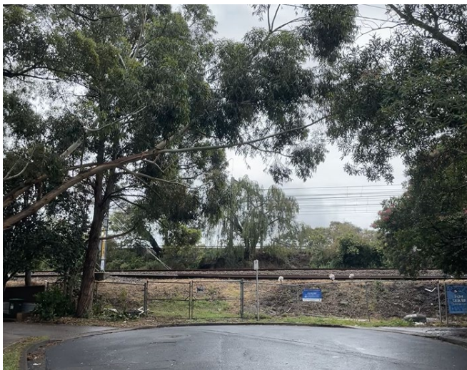
View of the rail corridor from Pilgrim Avenue to the north
