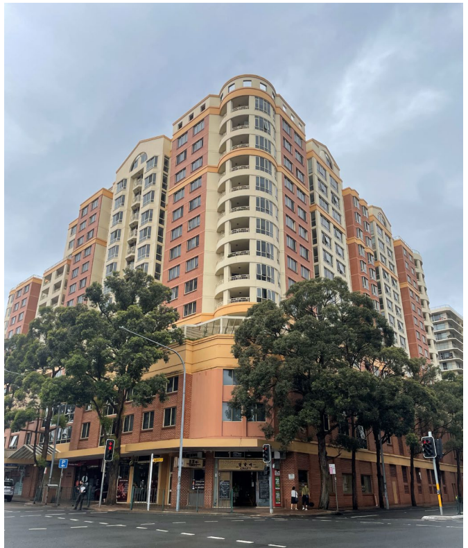
View of Regal Court Apartments from the corner of Raw Square and Albert Road to the south-east
