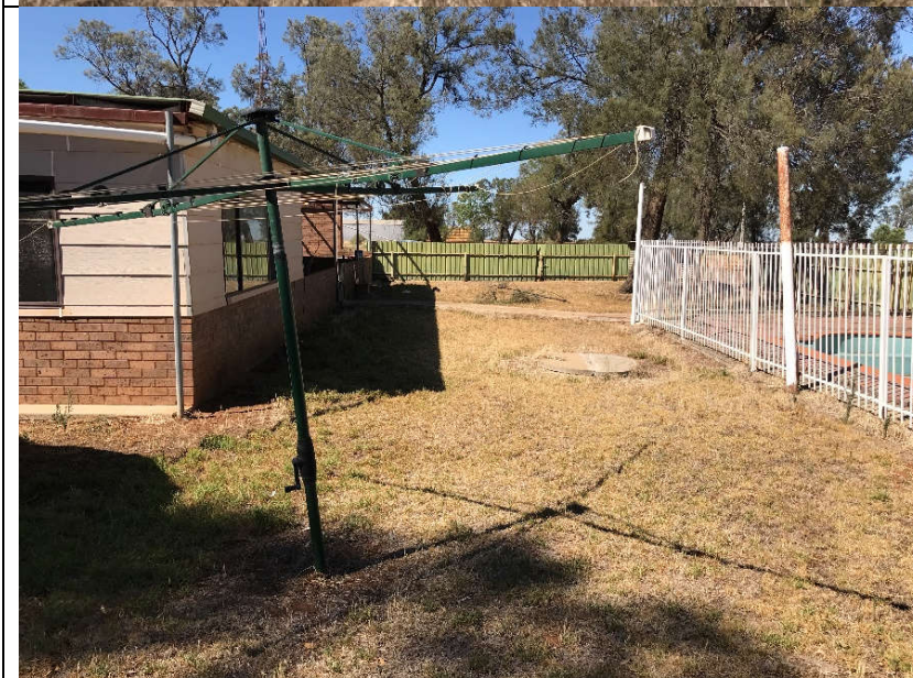
Plate 6 – Septic tank adjacent to the main house.
