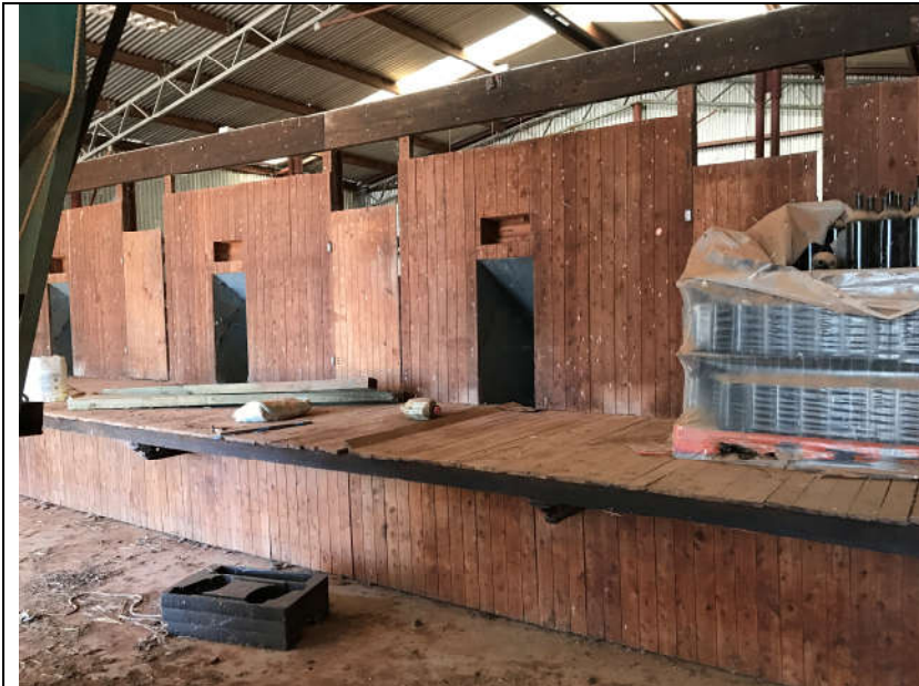
Plate 4 – Raised shearing board in the machinery and shearing shed.
