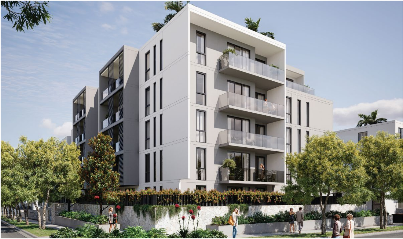
Picture 6 South Elevation
