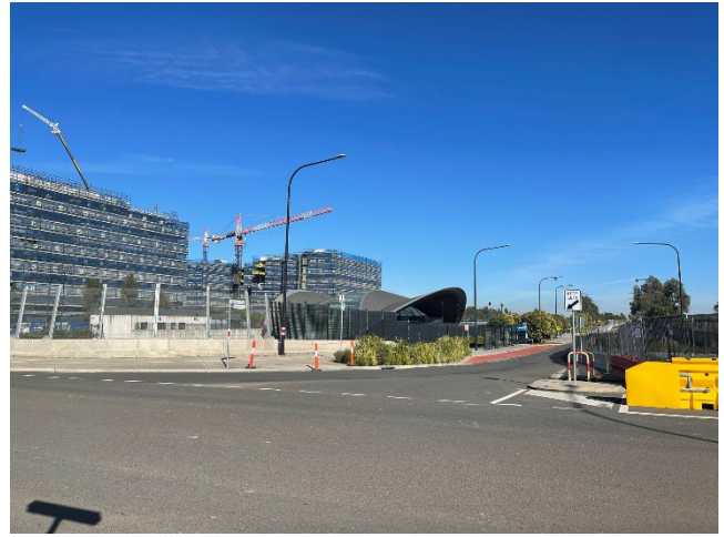
Picture 4 Tallawong Metro Station and emerging high-density development to the south (future Tallawong town centre)
