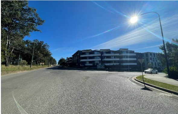
Figure 8 – Facing north along Cudgegong Road, near the intersection with Grassland Street.
