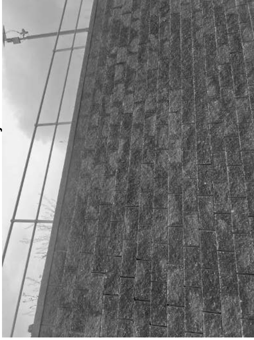
Southern Boundary Wall
