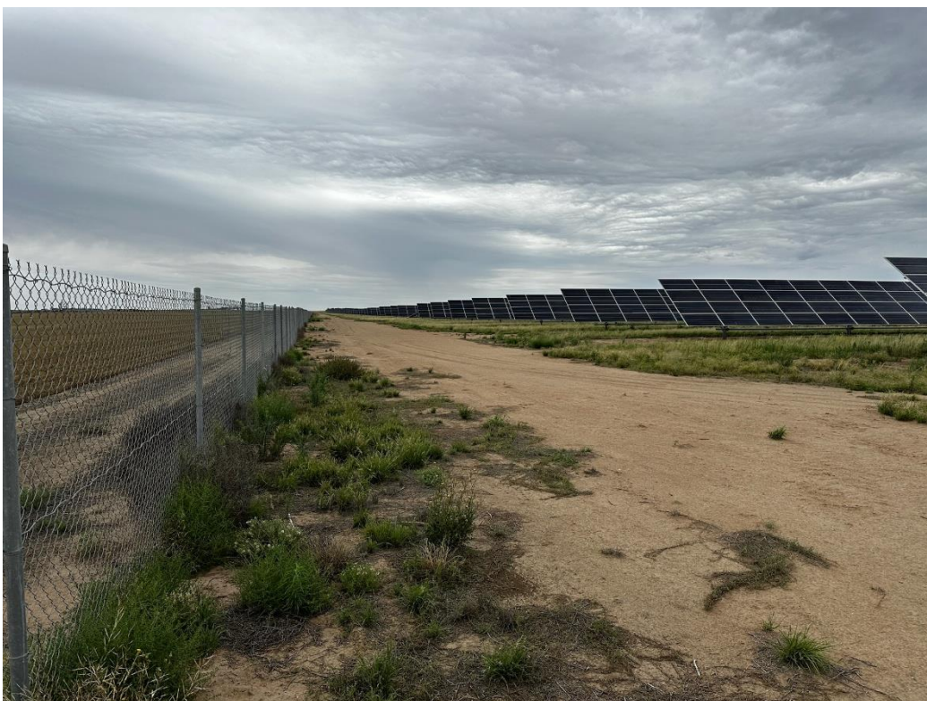
Photo 8: Solar farm and asset protection zone
