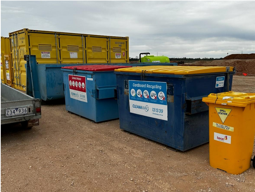
Photo 7: Waste and recycling bins, spill kit and bunded chemical storage container
