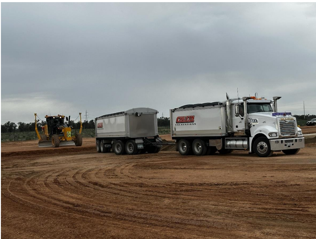
Photo 2: Spoil truck with dust covers
