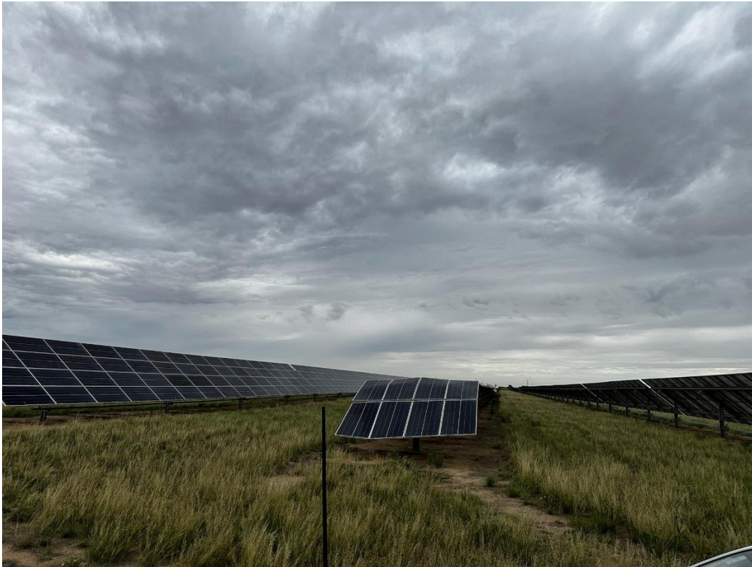
Photo 9: Solar farm rehabilitation
