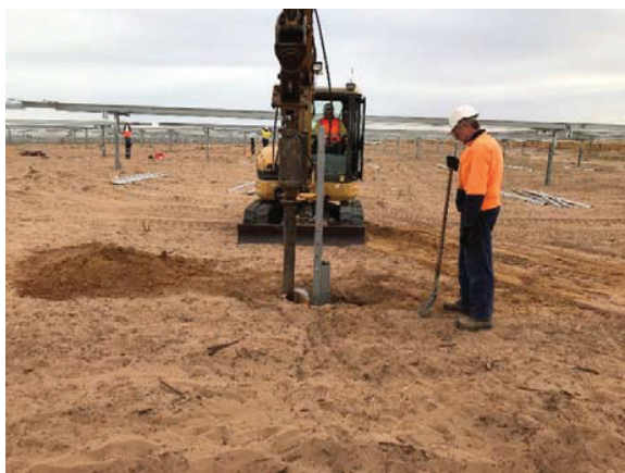
Plate 2.5 Example of post removal; view east
