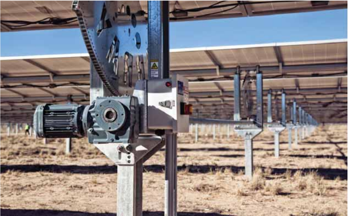
Photograph 4.2 Example of the steel frame structures used to support PV solar panels
