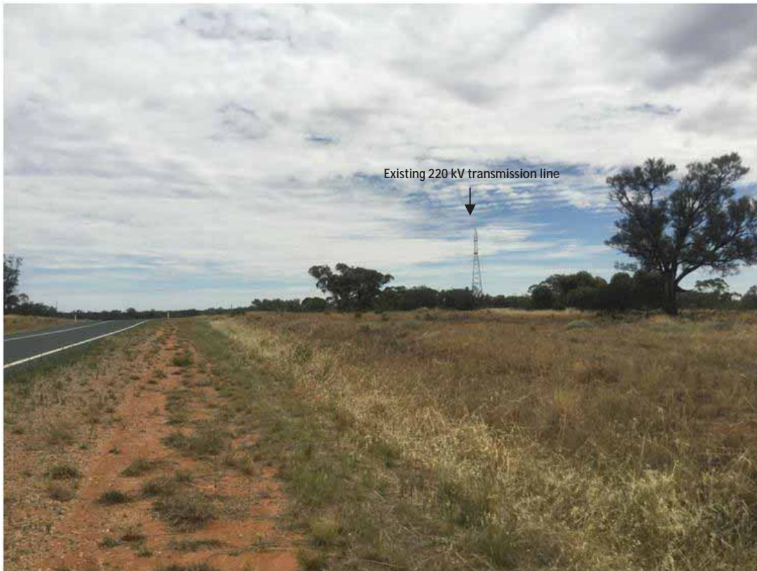
Photograph 5.8 Yanga Way north of the Balranald Substation looking south-west
