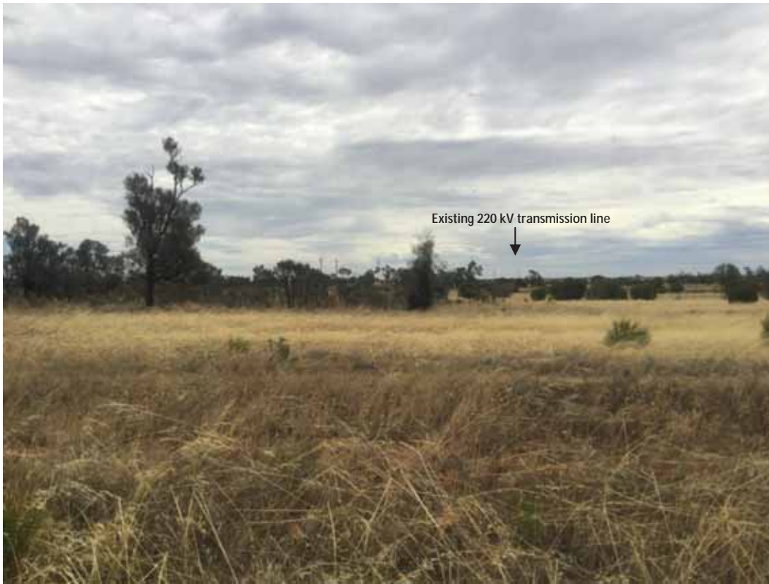
Photograph 5.6 Viewpoint 4 – Yanga Way north of the Balranald Substation looking west
