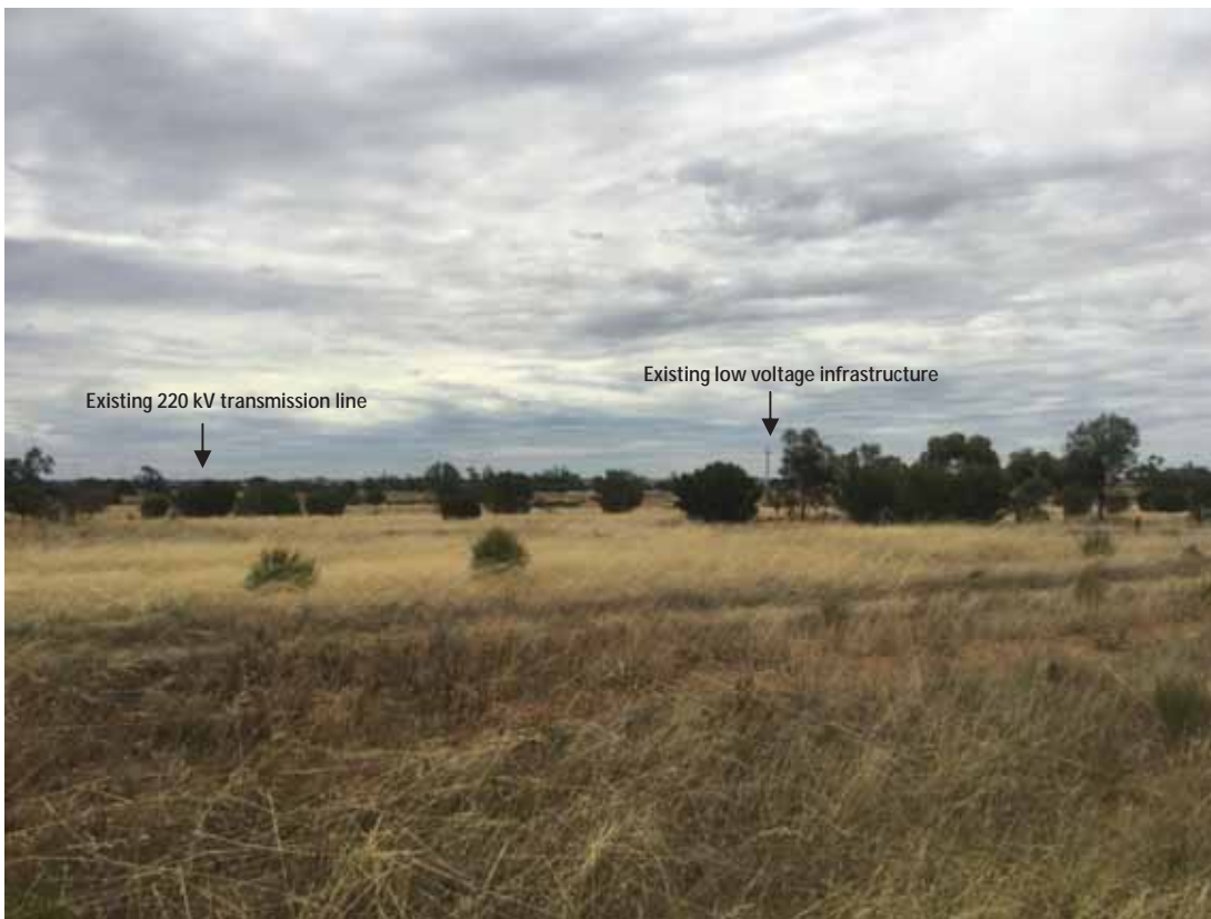
Photograph 5.7 Yanga Way north of the Balranald Substation looking north-west
