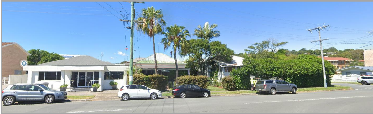
Figure 4: View of site from Florence Street
