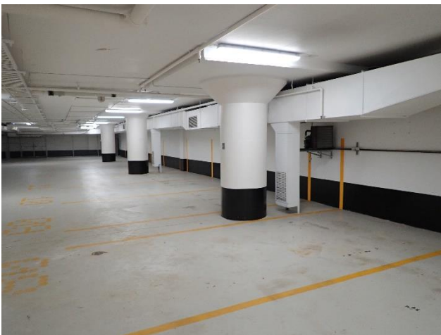
Figure 18 – Part of basement below building on corner of Forbes Street and William Street
