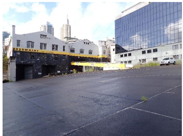
Figure 15 – View south-east of hardstand in north-western corner of subject area, bounded by Forbes Street and Judge Lane
