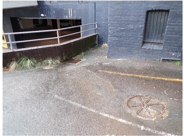
Figure 17 – Sewer manhole cover in south-eastern portion of hardstand area
