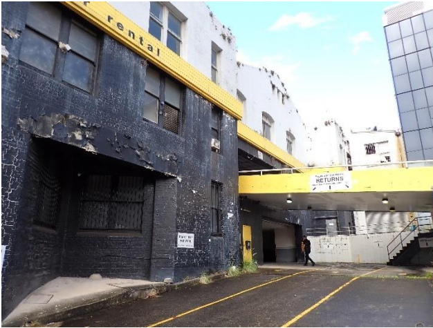
Figure 16 – Level change in eastern portion of hardstand area
