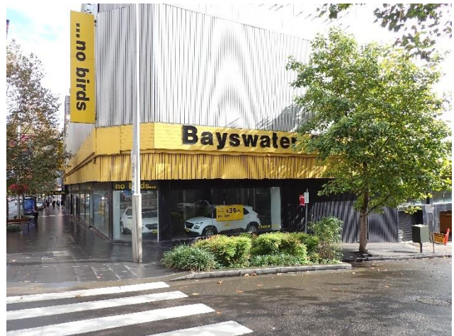
Figure 13 – View west of extant building at corner of Dowling Street and William Street, in south-eastern corner of subject area
