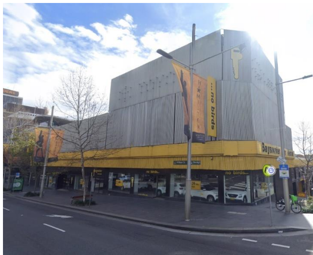
Picture 1: Site viewed from William Street
