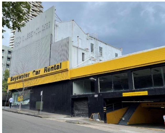
Picture 2: Site viewed from Dowling Street
