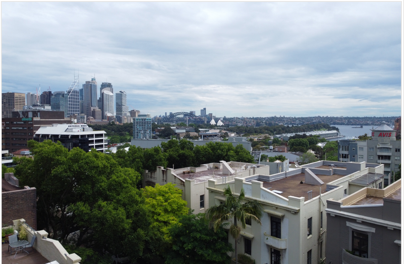
Existing site photo
