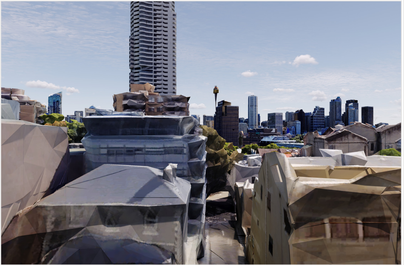
Existing site photo
