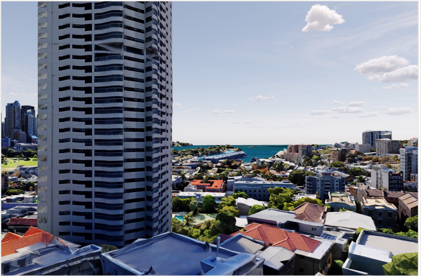
Existing site photo
