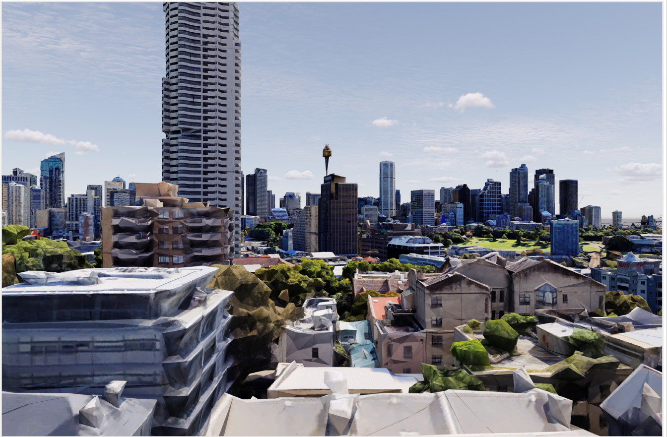
Existing site photo
