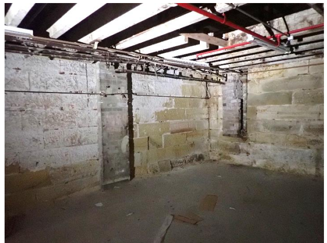
Figure 33 – Part of basement below building on corner of Darling Street and William Street
