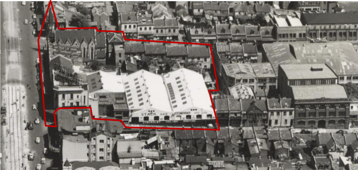
Figure 21 – “William Street branching out to Kings Cross, Victoria Street, etc., Sydney” [picture] / Frank Hurley (1950), showing the Stack and Company Pty Ltd building on Dowling Street, terrace houses on corner of William and Dowling Streets, terrace group on William Street, adjoining Wesleyan church and terrace houses on Forbes Street
