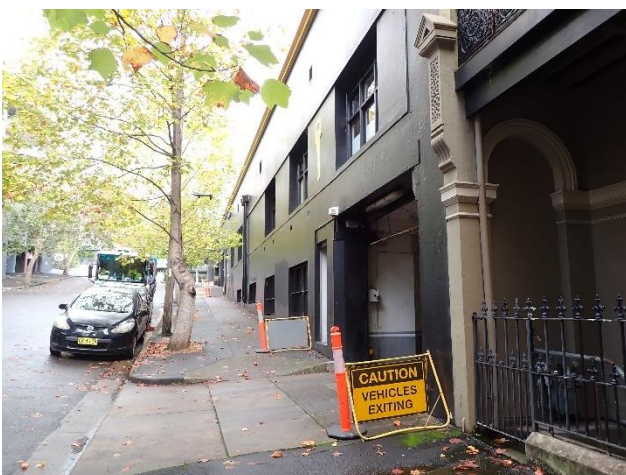
Figure 28 – View south of extant building fronting Dowling Street in north-eastern corner of subject area
