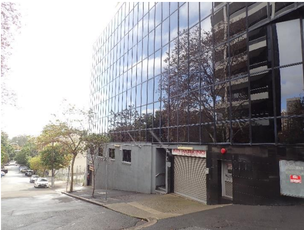
Figure 26 – View north of extant building at corner of Forbes Street and William Street, in south-western corner of subject area
