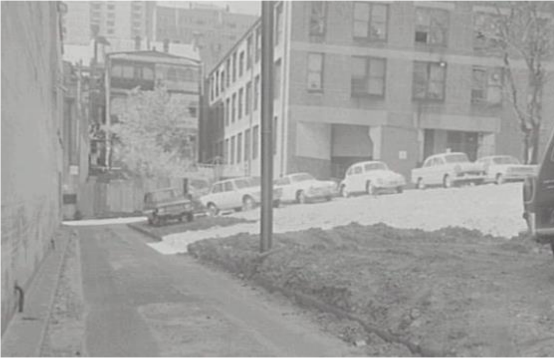
Figure 23 –View east along Judge Lane, Woolloomooloo, 1971. Post demolition of terraces along Forbes Street
