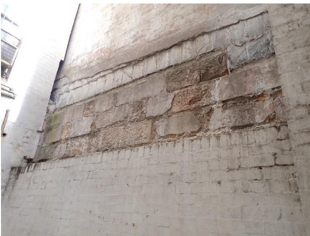
Figure 34 – View of sandstone wall at the rear side of No. 172 William Street
