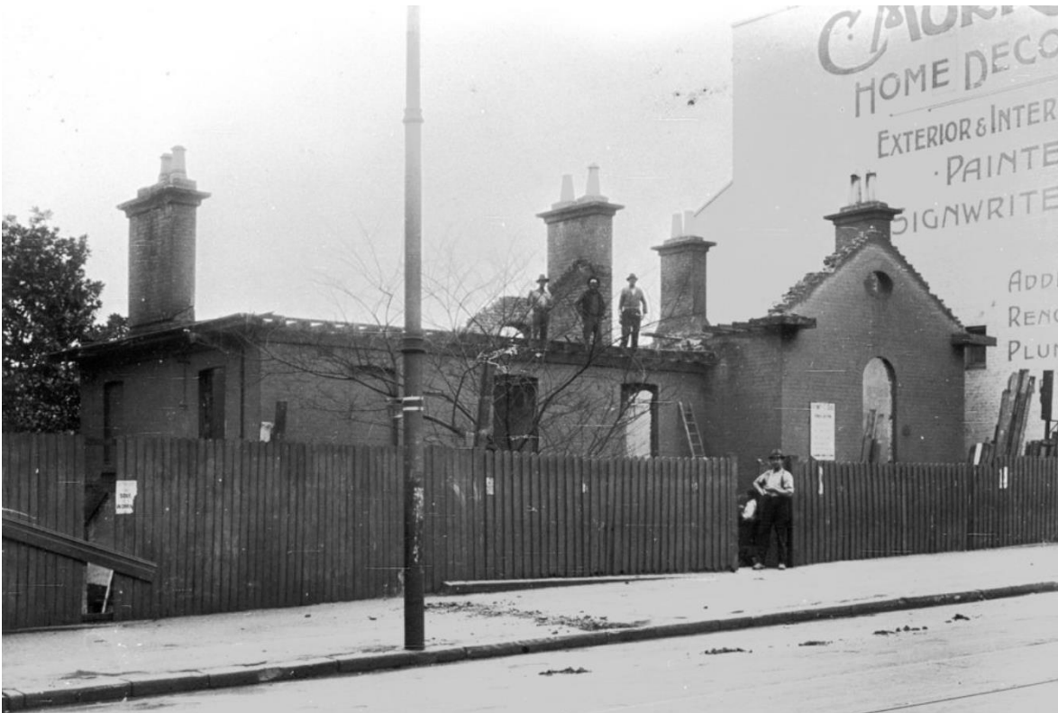
Figure 18 – 1921 Demolition of Ailanthus College
