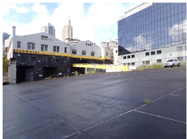
Figure 29 – View south-east of hardstand in north-western corner of subject area, bounded by Forbes Street and Judge Lane
