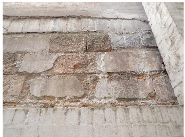
Figure 35 – Detail view of sandstone wall at the rear side of No. 172 William Street
