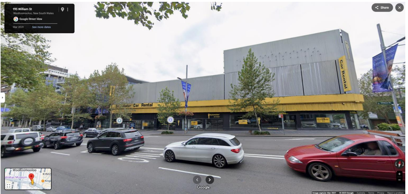
Figure 10: A view of the study area from the south (on William Street), showing the two commercial buildings present.
