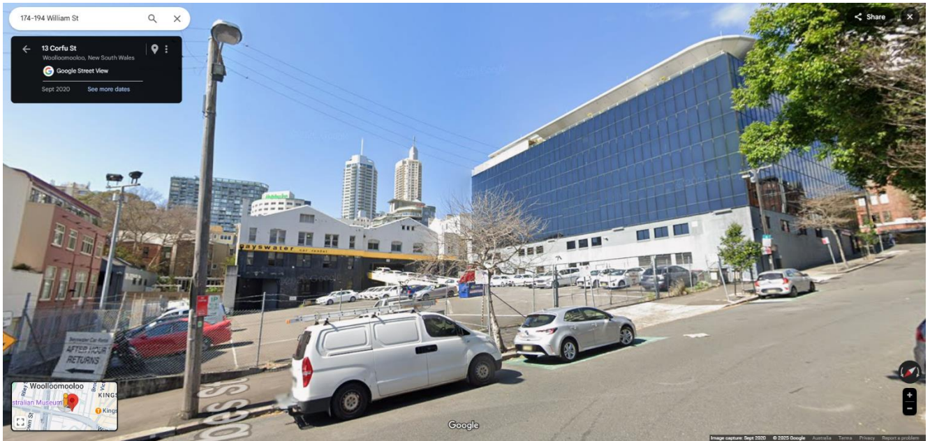
Figure 11: A view of the study area from the west (on Forbes Street).
