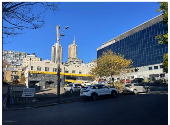
Picture 6 Rear of site, looking south-east from Forbes Street
