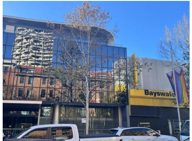
Picture 4 Site frontage along William Street, looking north
