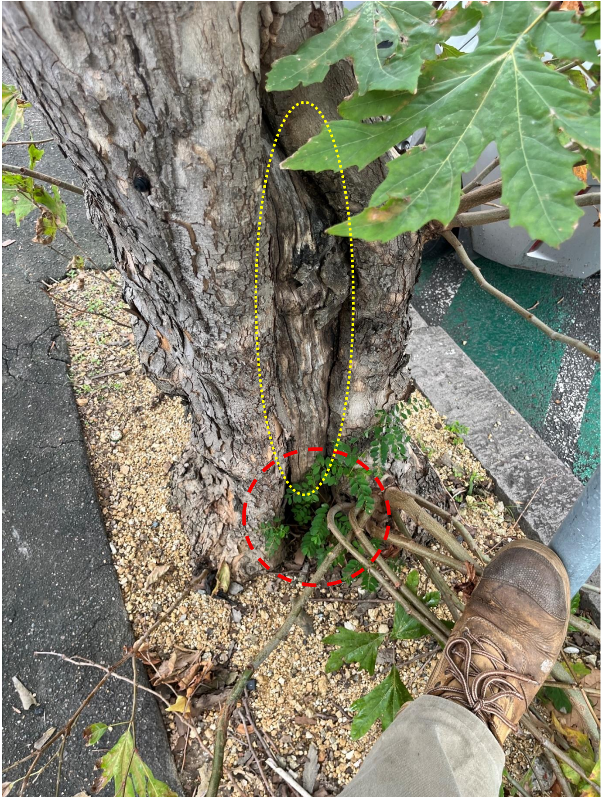
Tree 1 – Platanus x hybrida – London Plane Tree - Cavity at the base of the tree and cambium damage is present
