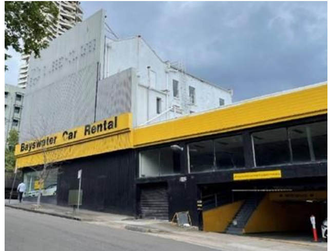
Picture 2: Site viewed from Dowling Street
