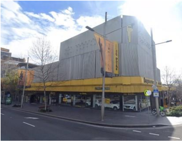
Picture 1: Site viewed from William Street
