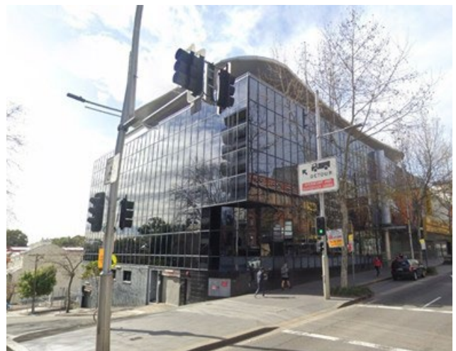
Picture 4: Site viewed from the corner of William and Forbes streets
