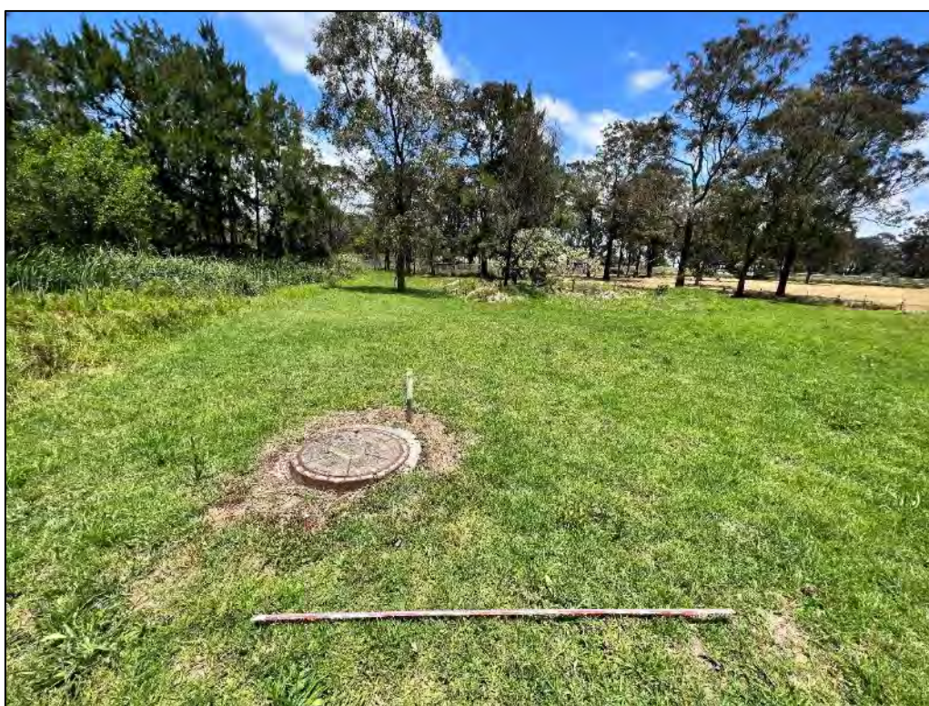
Plate 11: Looking south east within the Sydney Water easement and proposed bridge crossing location.
