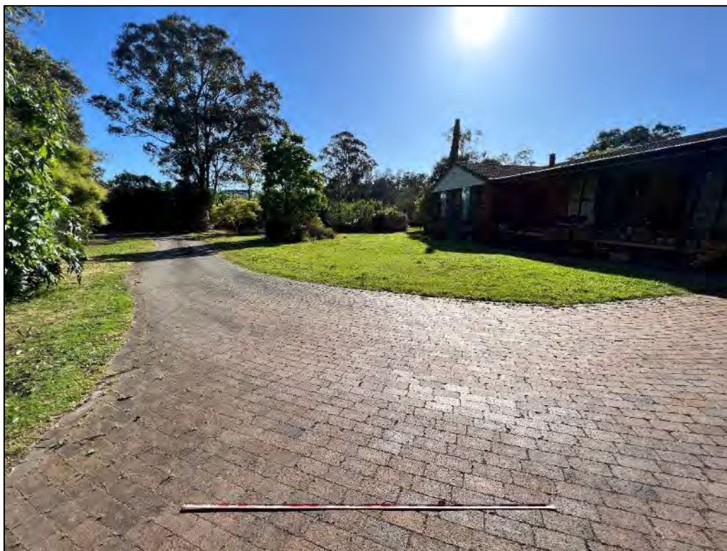
Plate 6: Looking east across the front of the main residence.
